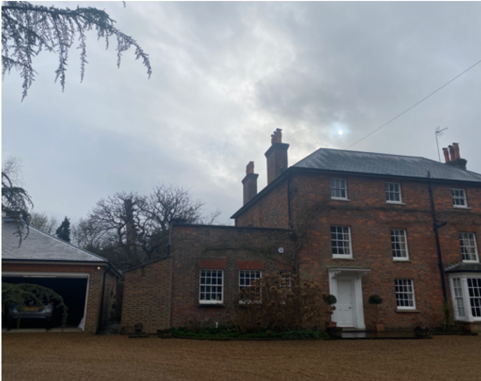
IMAGE OF ROOF TO FRONT ELEVATION. The roofs prevent view of the proposed antenna
