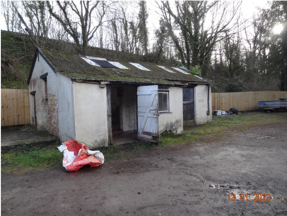
View of former dairy/cowshed from yard area – 13.01.2023.
