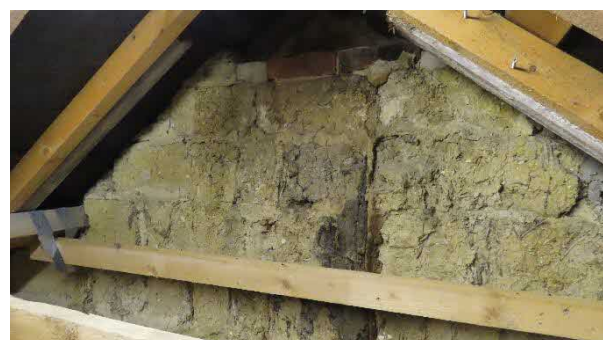
End gable in older section of the roof
