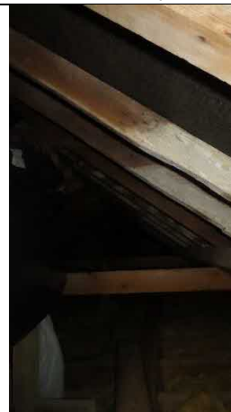
Roof space older section
