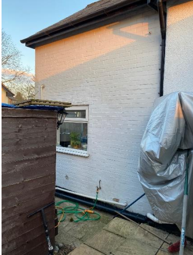
Existing white painted brick
