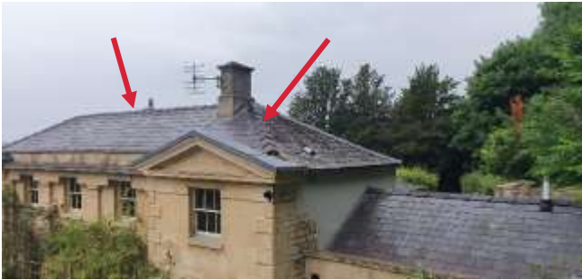
Figure 4 – Eastern elevation with bat emergence points (arrowed)
