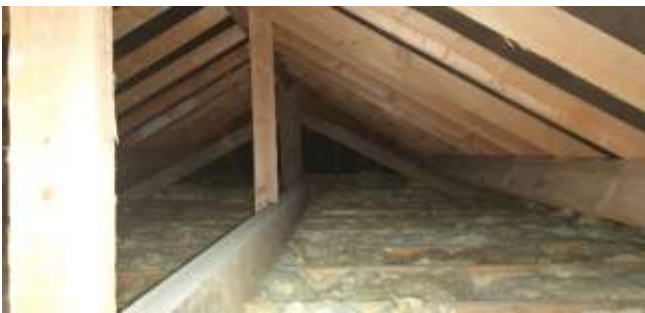
Figure 6 – Internal view of main house roof space
