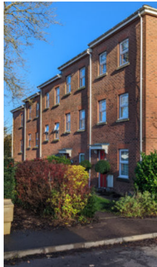
Three storey terrace house to the south east of the site.
