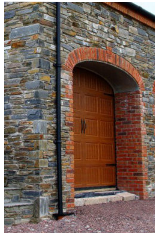
Brick arch with stone work.
