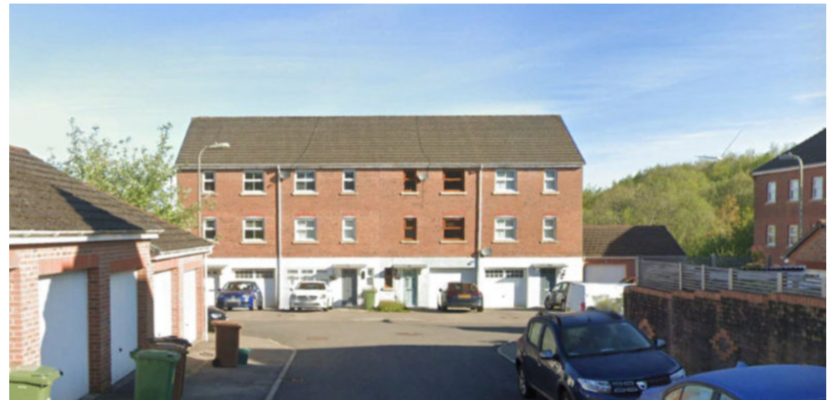
View 4 - View north down Blacksmith Close. (3 storey town houses)
