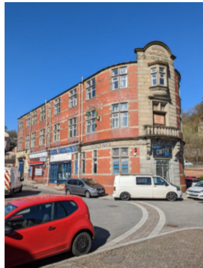
Elevational Approach Institute Buildings, Crumlin replicates a similar approach using horizontal banding, stone window surround and stone pediments to subdivide its brick elevations.
