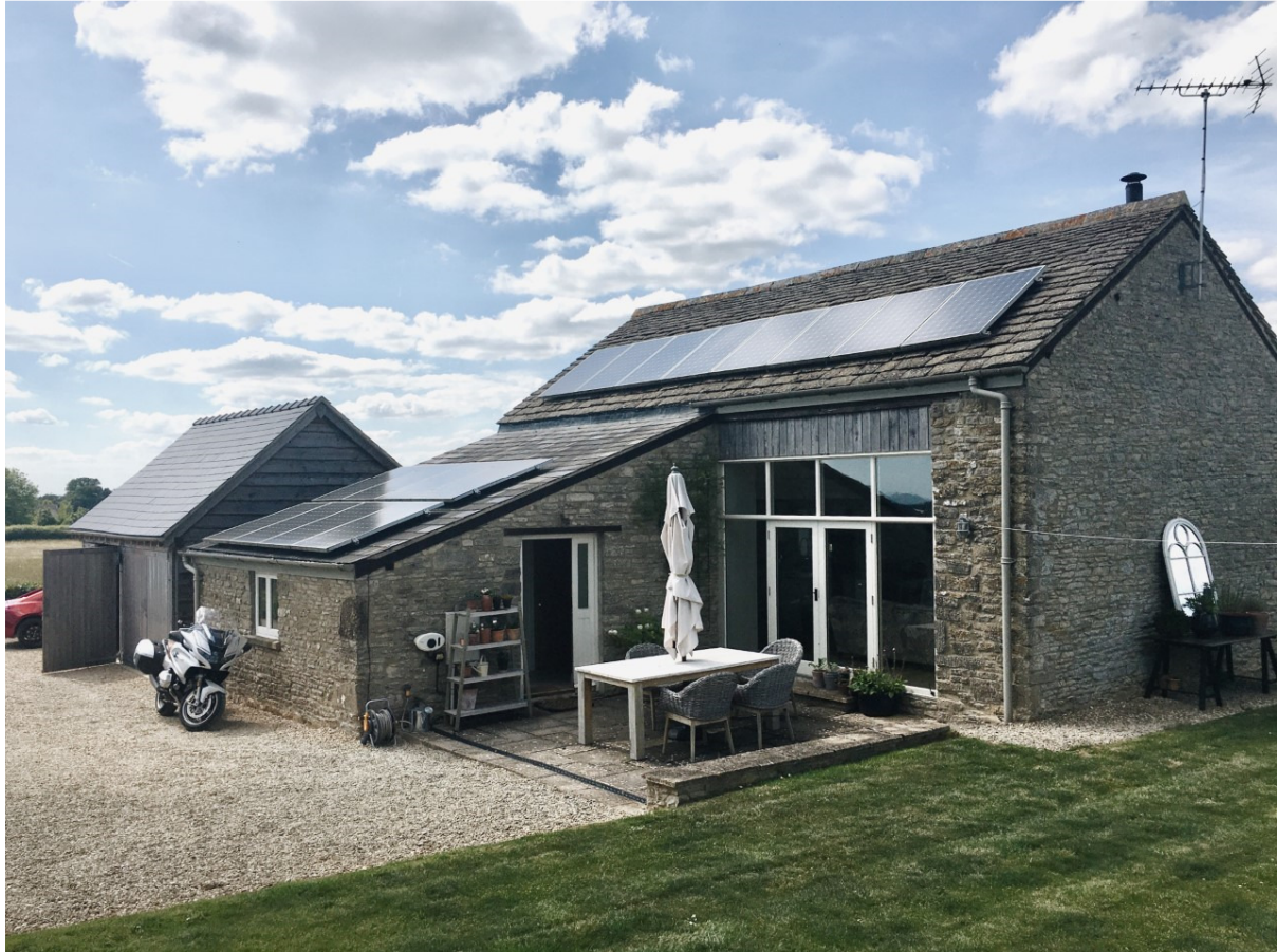
Figure 2 – Garden view of the applicants dwelling and garage (south elevation)
