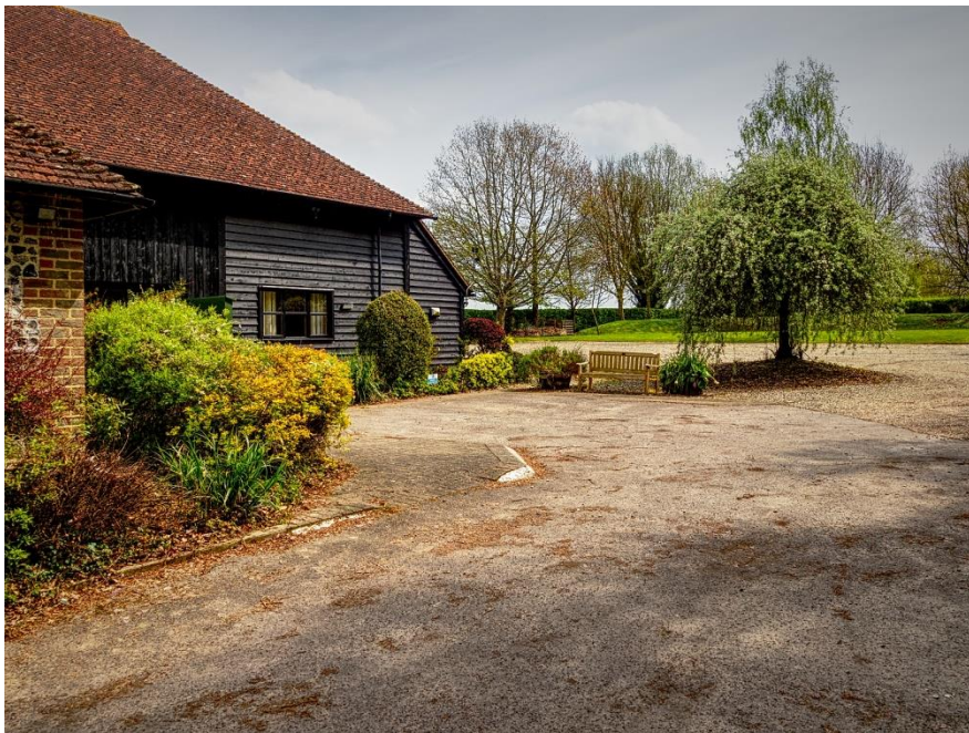
Figure 4 - View towards location of proposed extension
