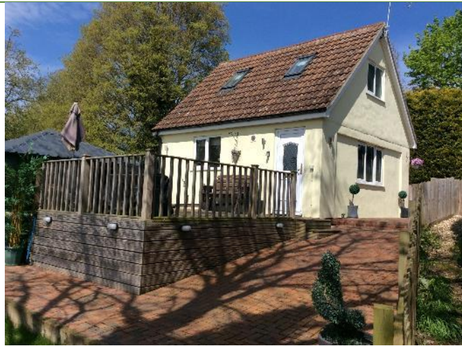
Photograph 1. Existing dwelling south and east elevations.
