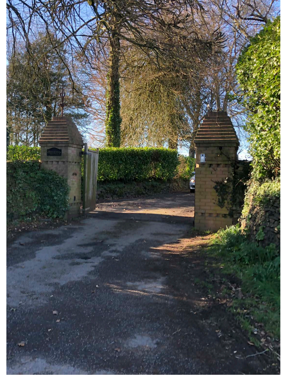
Photo of existing entrance gate piers.
