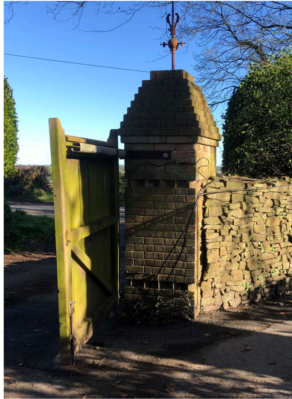
Photo of existing entrance gate pier.
