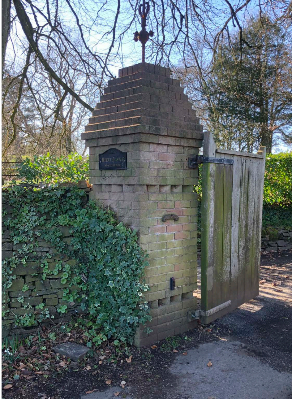
Photo of existing entrance gate pier.
