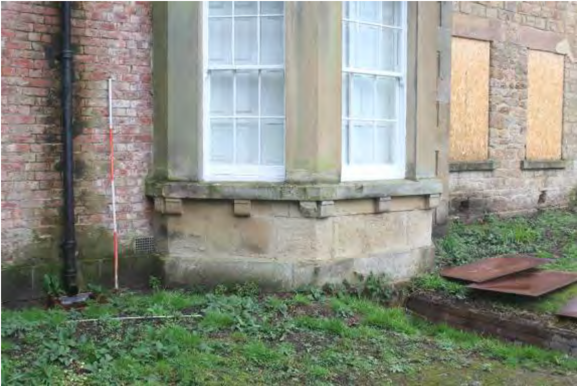
Photo 16. Ventilation grille to LHS of bay (adjacent to ranging rod)
