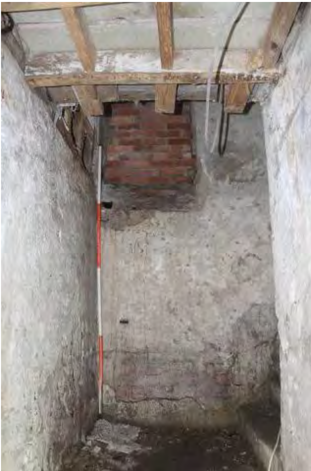
Photo 1. Opening with modern blocking at N. end of passage. Base of steps to right
