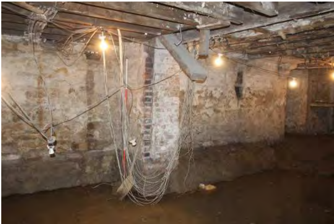
Photo 15. Surviving jamb of doorway broken through earlier wall (now largely removed). Note ventilation slot at high level to L. and "tide mark" indicating original floor level in both cellars
