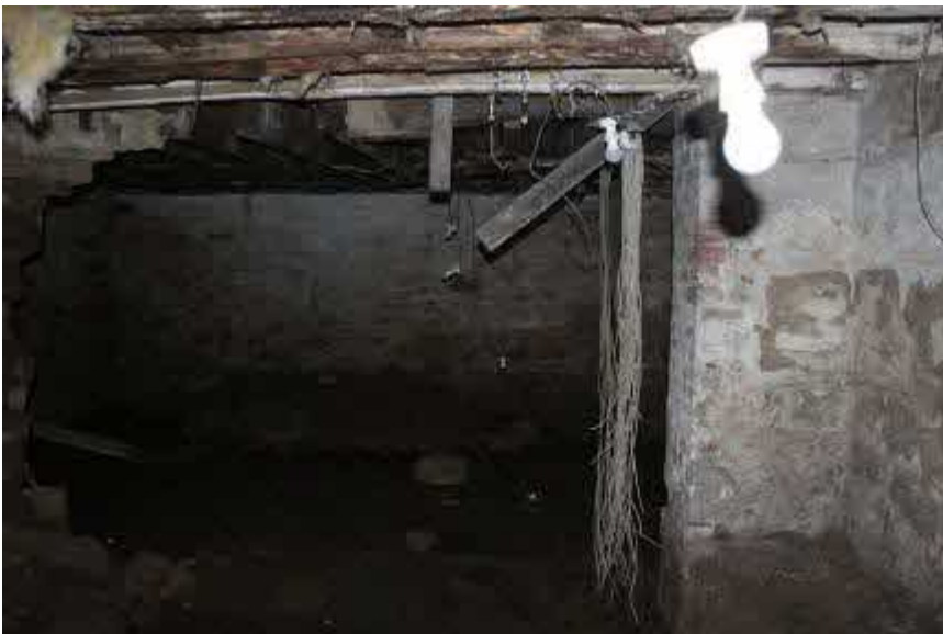
N side of doorway between 1840's cellar and 1880's cellar beyond. All of dividing wall to L removed leaving joists hanging
