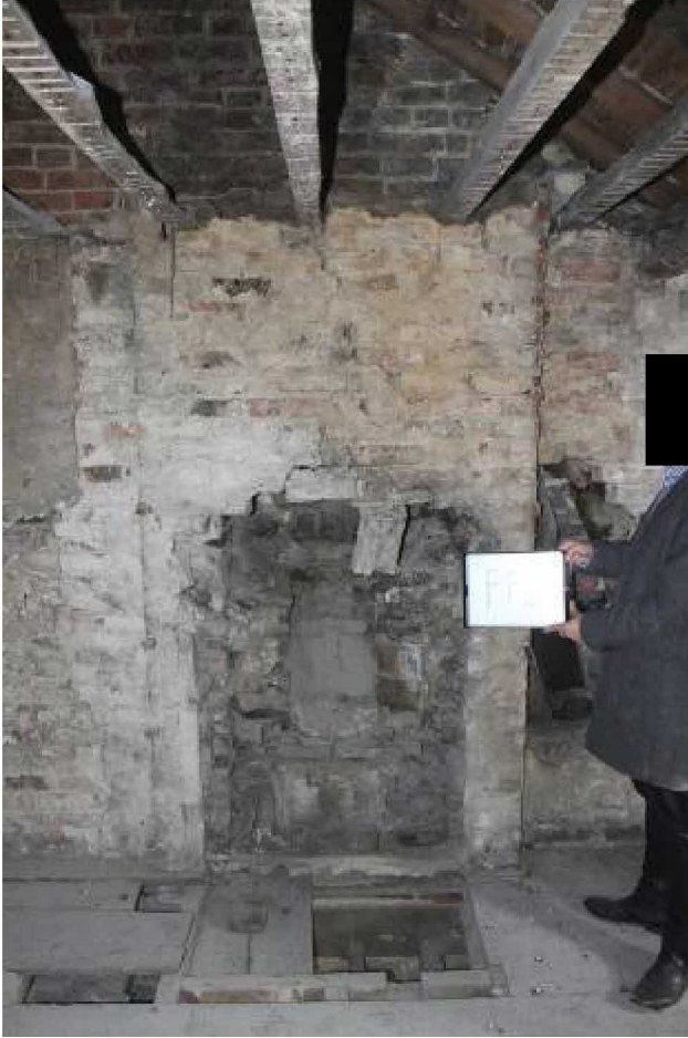
FP12 ?C18 hob grate here orig. , as FP13, but modified for C19 CI fireplace (fixings and outline).
