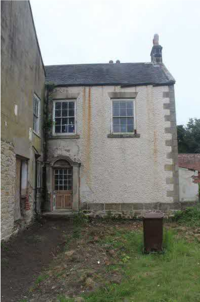
S elevation of early C18 house. Ground in foreground has been excavated in anticipation of earlier proposed linking conservatory
