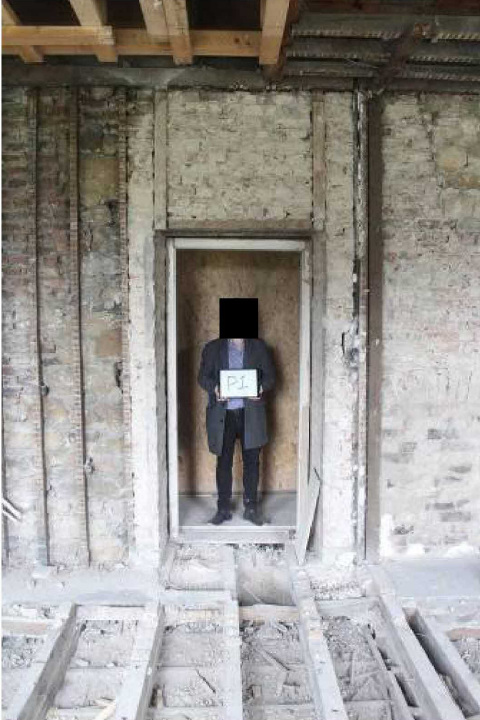
Bedroom side of D28, to be blocked (P1). Note blocked FP to R. C20 western bathroom partition in front of it
