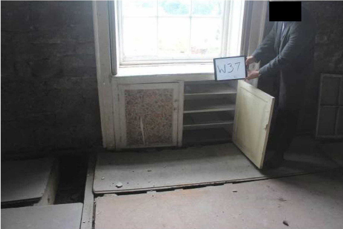
Cupboard below W37
