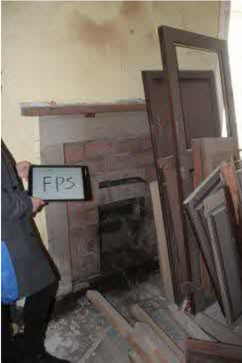
FP5 modern brick insert into earlier fireplace
