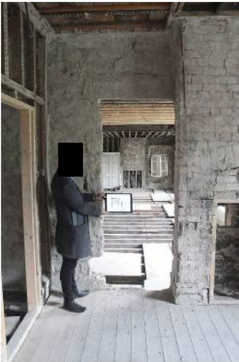
Breach cut through to S range
