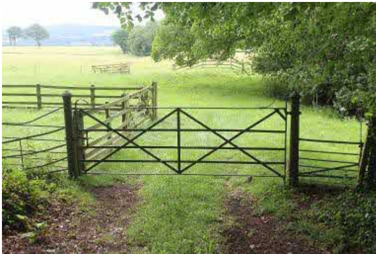
Victorian Cast Iron posts and wrought iron gate leading into parkland from the drive
