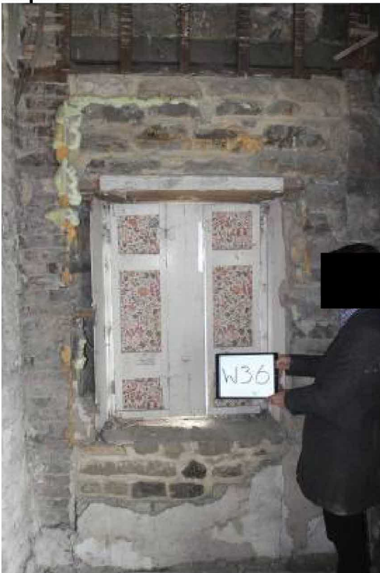
W36. C18 window (matching W35) reduced in C20. Shutters re-used?
