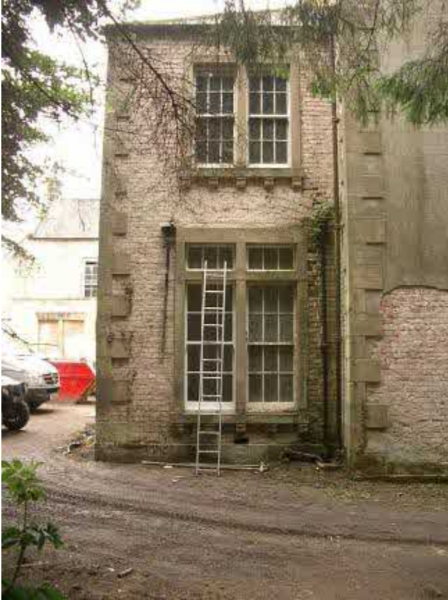
NW corner. 1880s addition. Large W21 GF, W44 above
