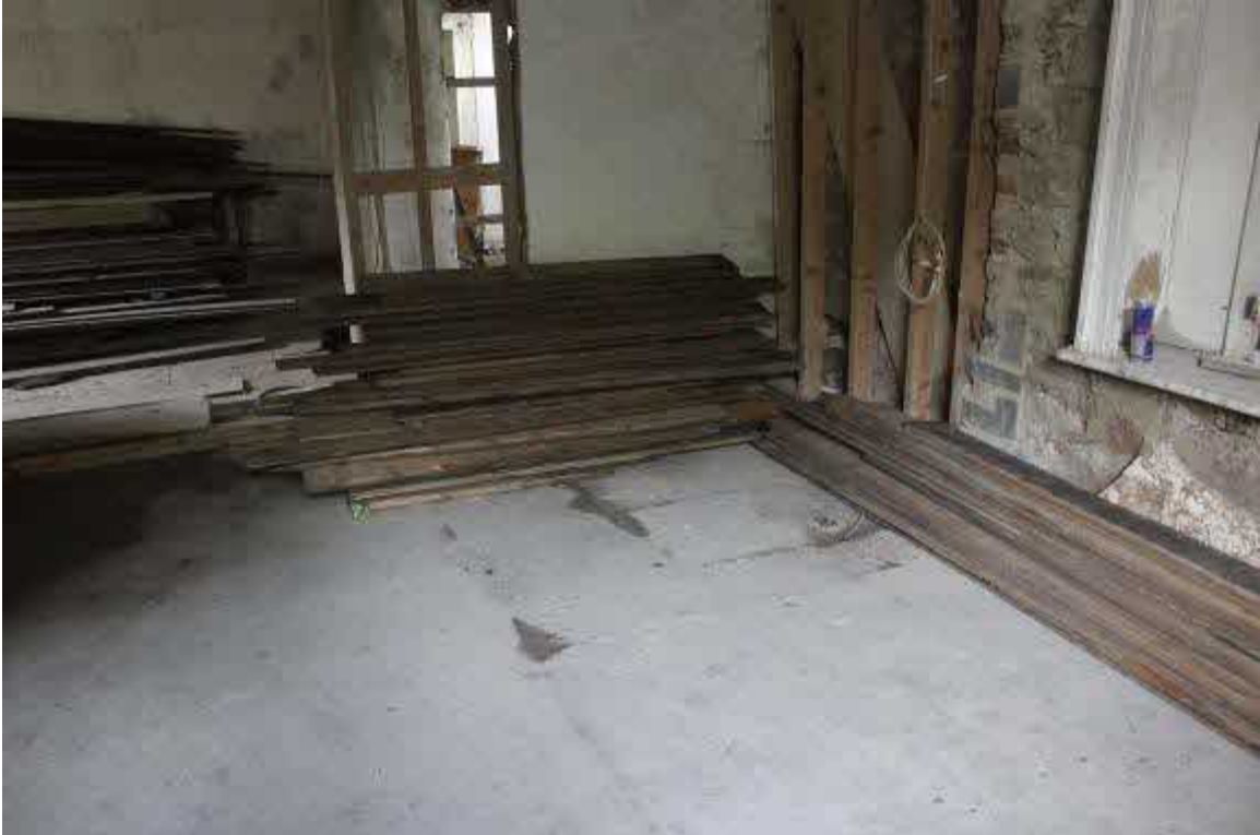
Footprint of former Plate Store shown on 1987 plan, removed when modern kitchen made. Beyond the partition was a pantry and passage
