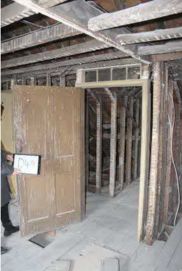
D44 corridor side with fan light over. Note hewn top sides to ceiling timbers
