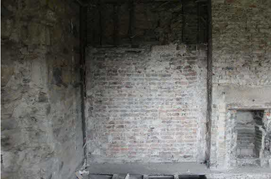
Brickwork panel infilling former doorway (now corridor cupboard served by D22) on N wall to L of FP8
