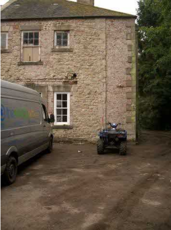
Cut back return of lost NW range. Sockets for previous FF joists above embedded timber. 1880s brick addition to R.
