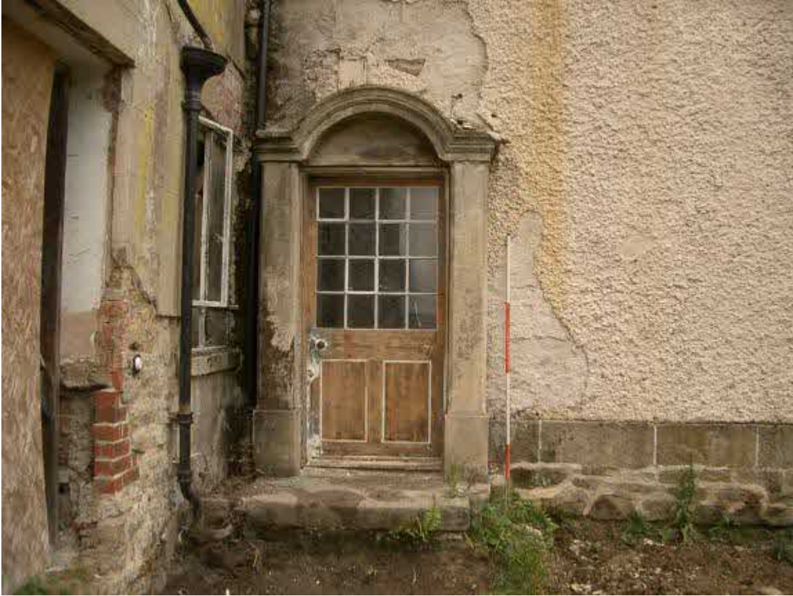
Detail of early C18 doorway in shallow stone porch. The glazing in the door is a late modification. The previous excavation has left thresholds and base plinth "perched".
