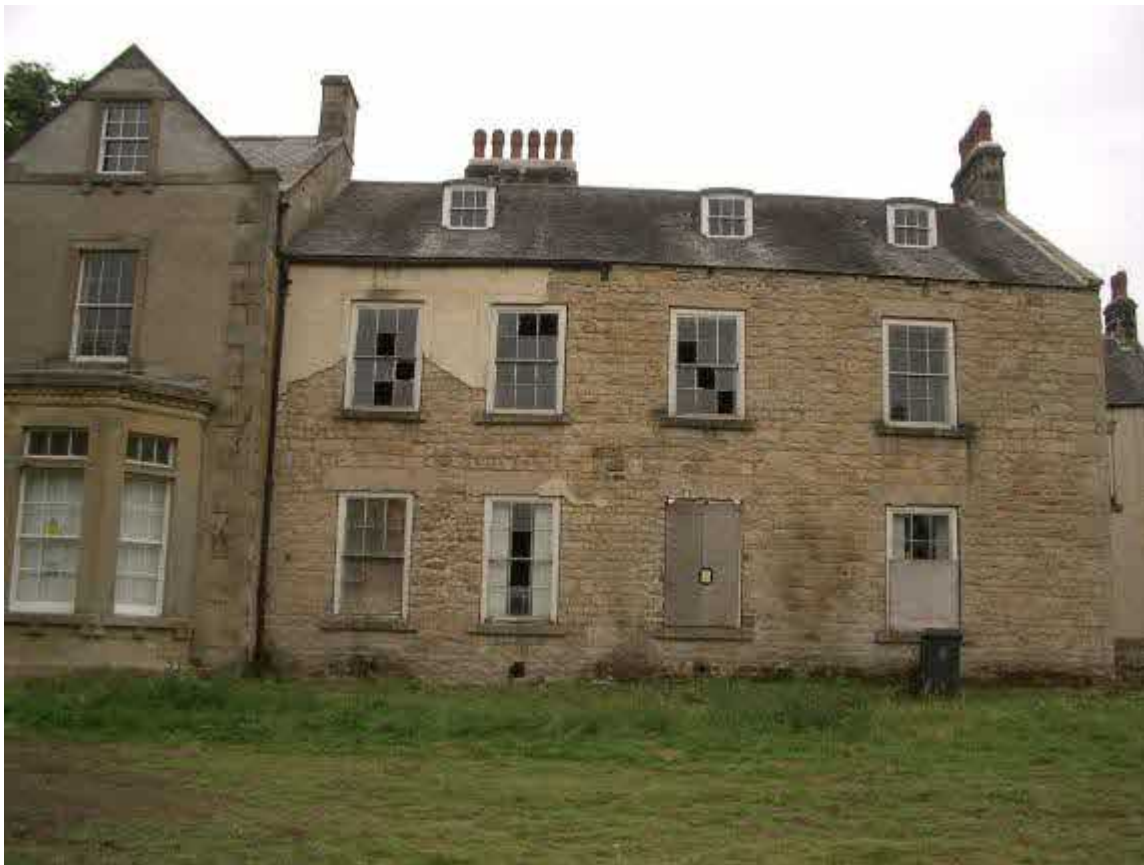
The south range of the late C18/early C19 house
