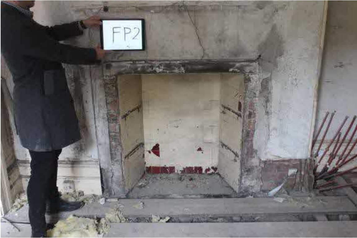
FP2 1930's tiled insert to original construction hearth? The pipework to R is from an attempted modern underfloor heating installation. Some skirting surviving
