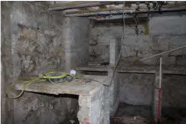
From entrance passage looking ENE
