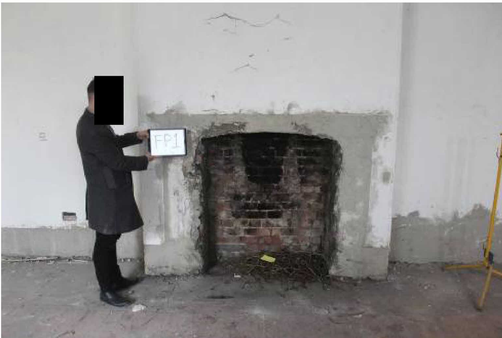
FP1 removed. Scar gives an idea of dimensions
