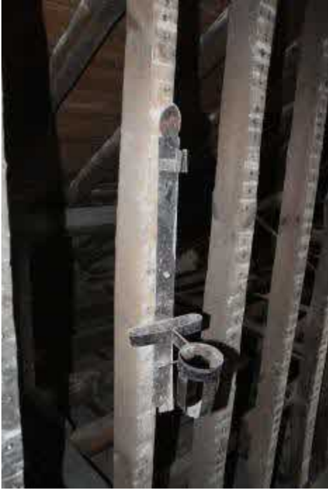
Early fire extinguisher bracket In corridor adjacent D48
