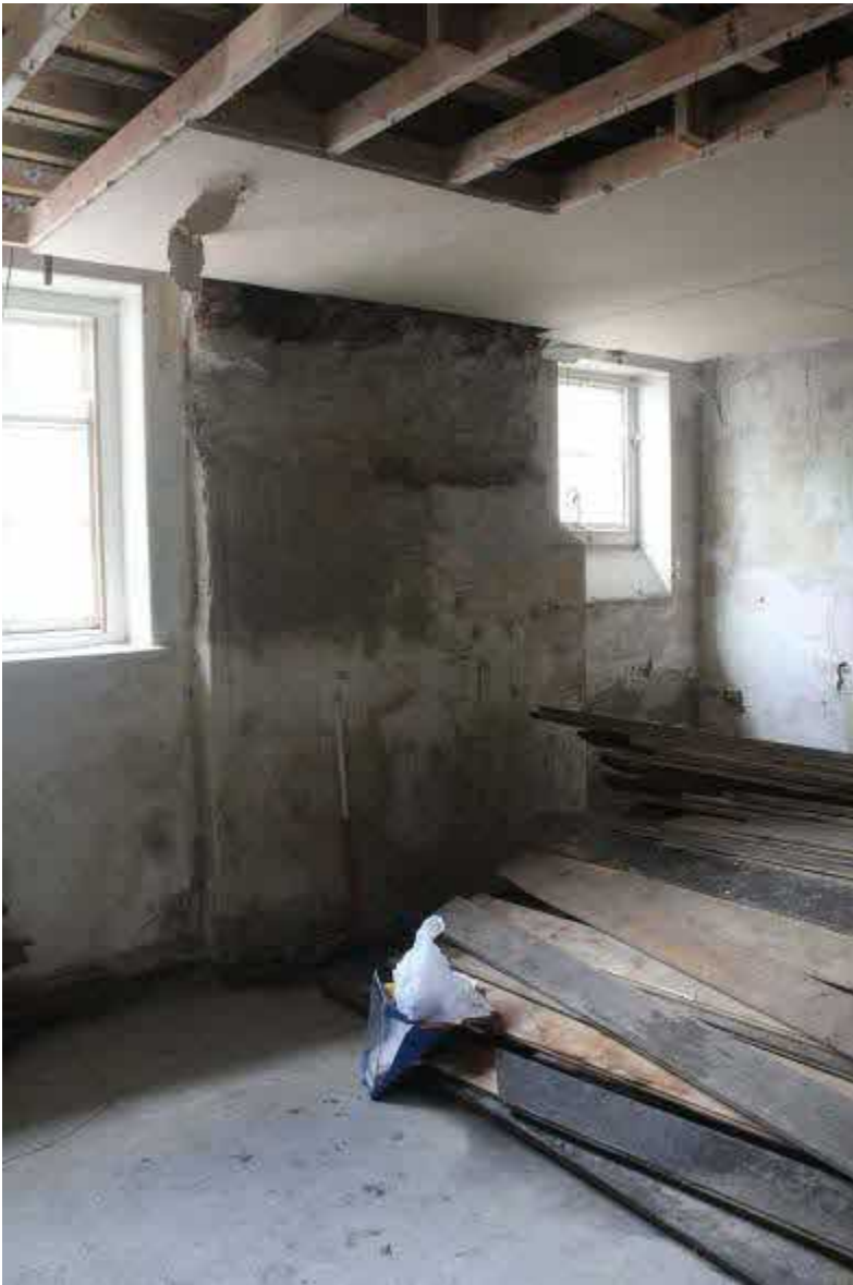
Blocked fireplace on N wall of former billiards room Between W6 (L) and W7 (R) flue above to left
