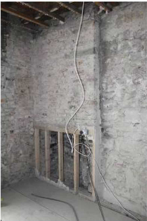
Fireplace in SE corner
