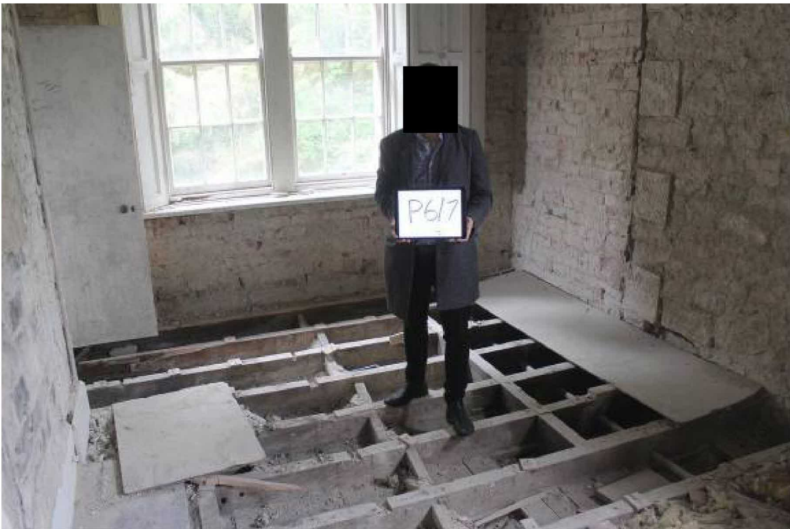
Proposals 6 and 7, as is. Note the junction of the 1880's build in brick and the earlier projecting quoins on the N wall, to R of figure
