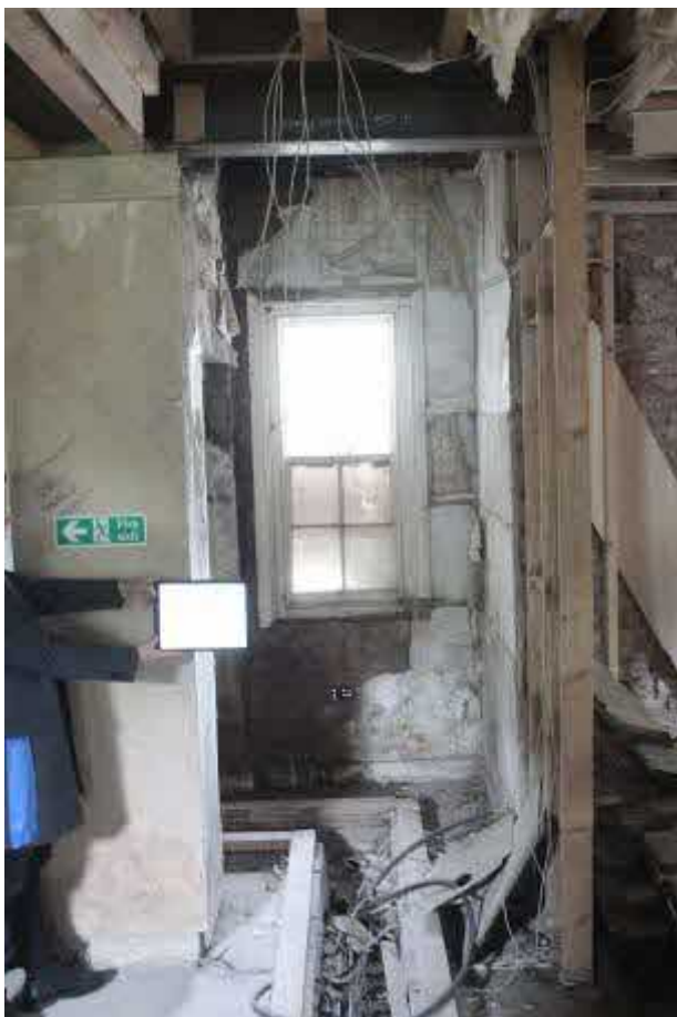
Location for P19, looking west. Note RSJ above and floor duct from previous works
