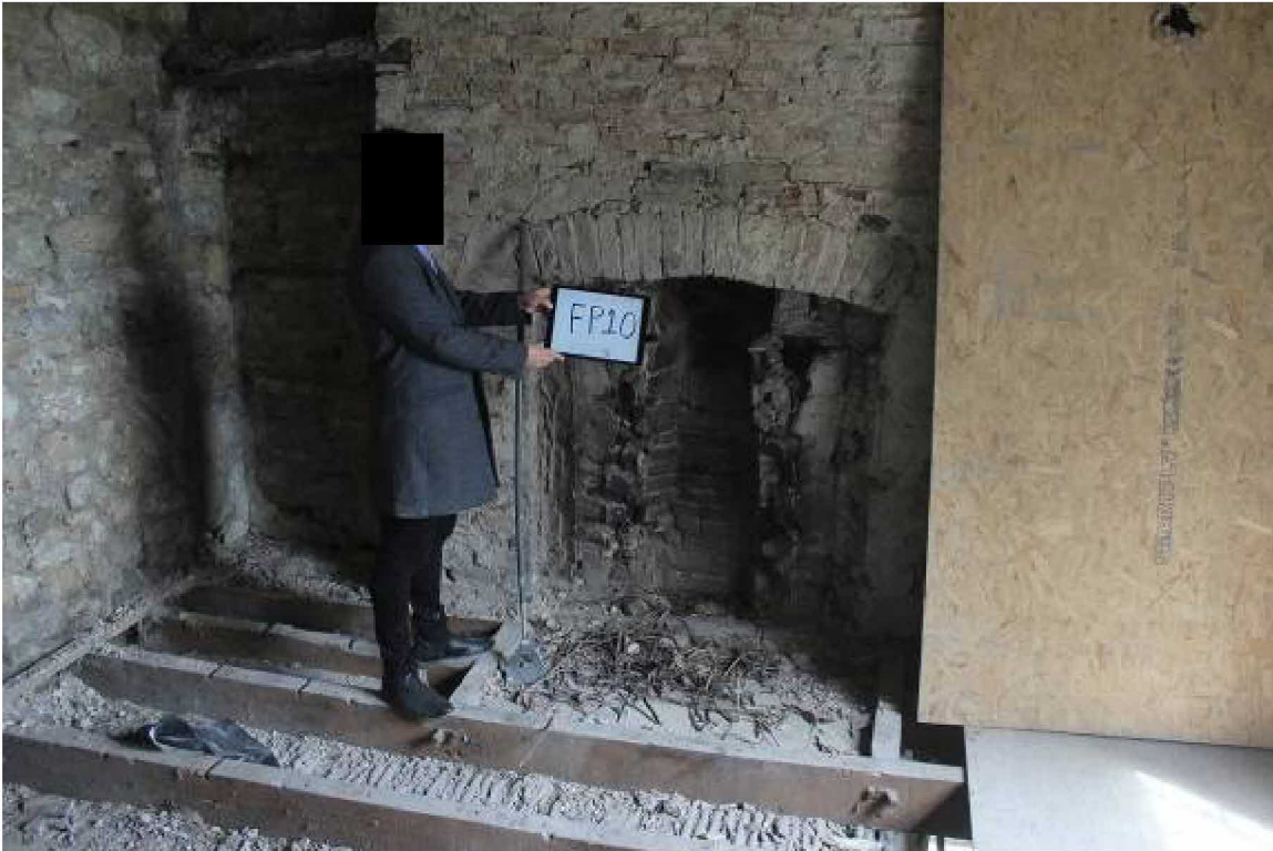
FP10 Cupboard with shelves to L (D38) removed
