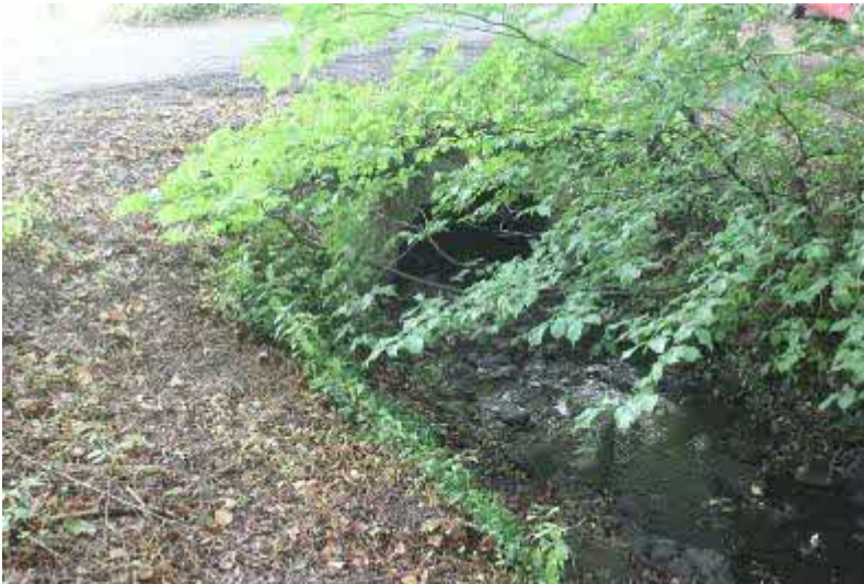
Brick culvert beneath drive
