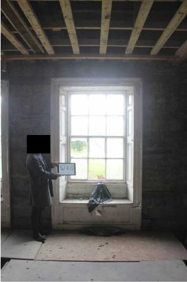
W 40 with shutters and window seat below
