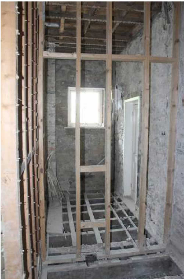
Looking N into northern bathroom. Inserted W30 and high level cistern suggest 1930s alteration
