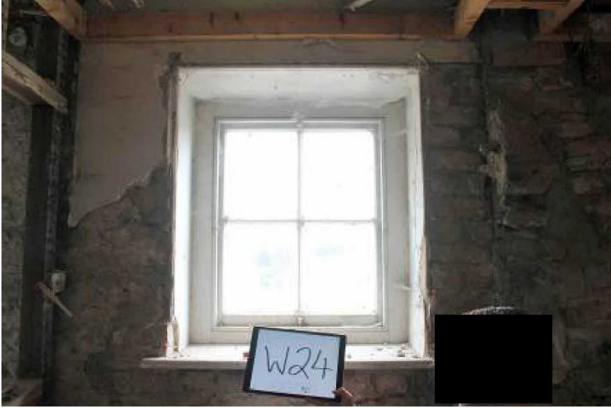
W24 1930's insert, as W22. Note stub of return of earlier late C18/early C19 range to R.
