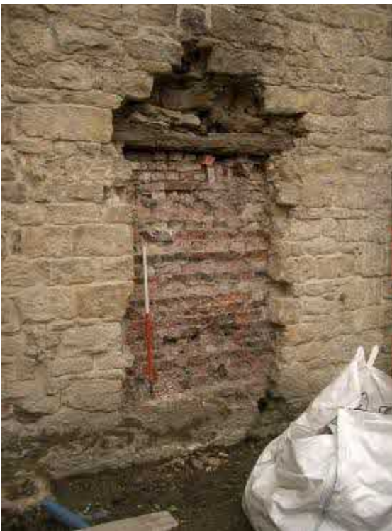
Blocked doorway (C18/early C19 bricks) in older rubble walling
