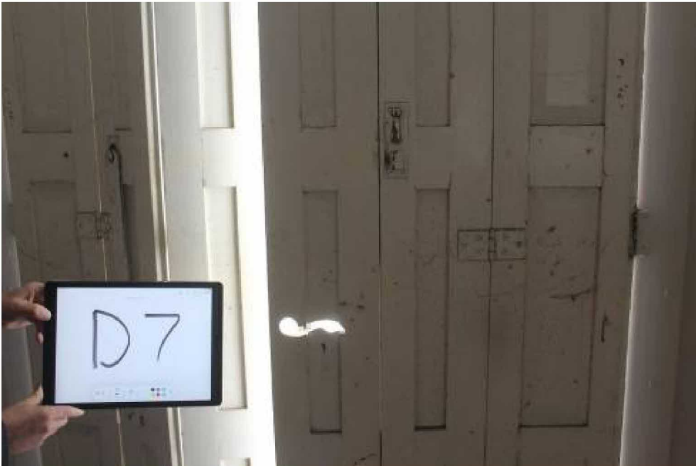
Detail of shutters deployed for D7. “push button” catch for locking bar and neat cut out for opening (no projecting knob)
