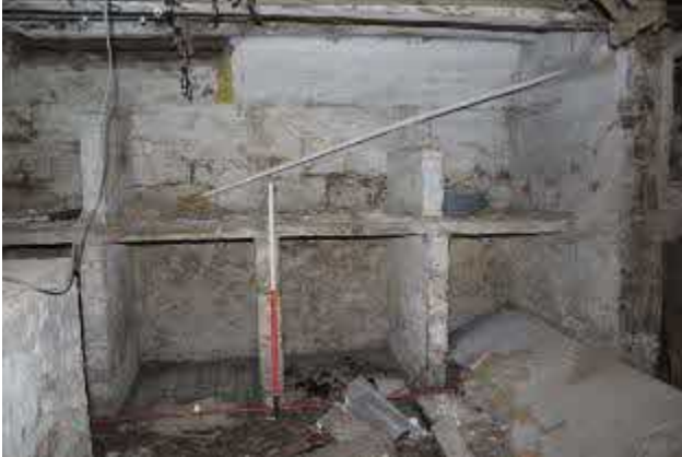
Looking E to wine bins. N.B. brick floor
