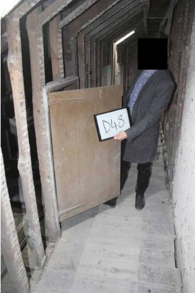
First of 3 low access doors to storage area. Earlier blacksmith made hinges. Note bolted strap on hanger to RHS doorway
