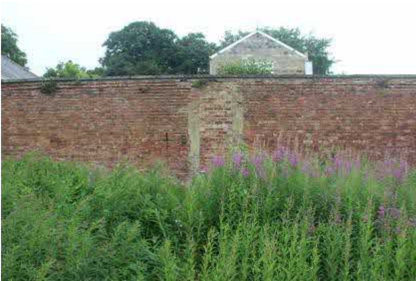
Blocked doorway from stable yard behind
