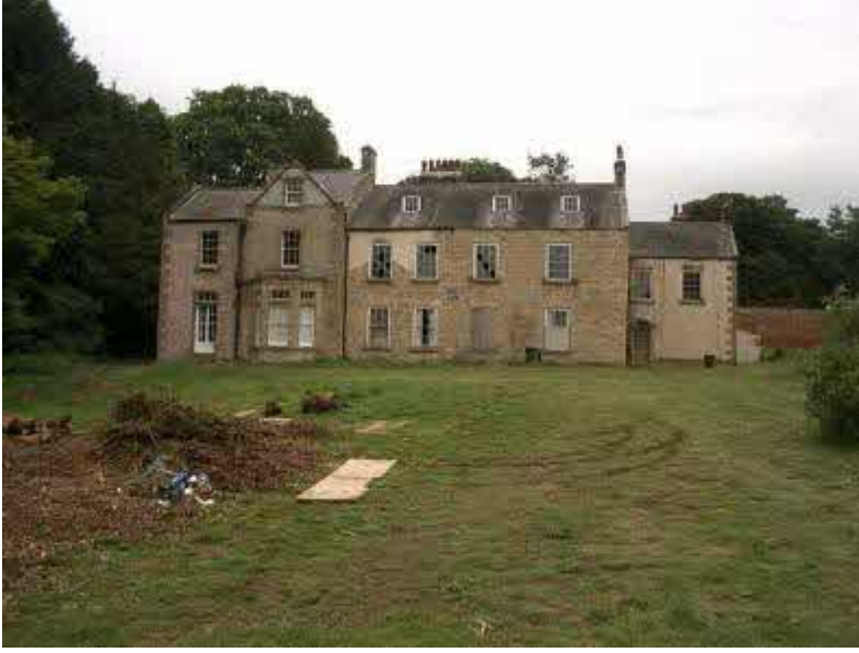
House from S edge of pleasure ground, looking North
