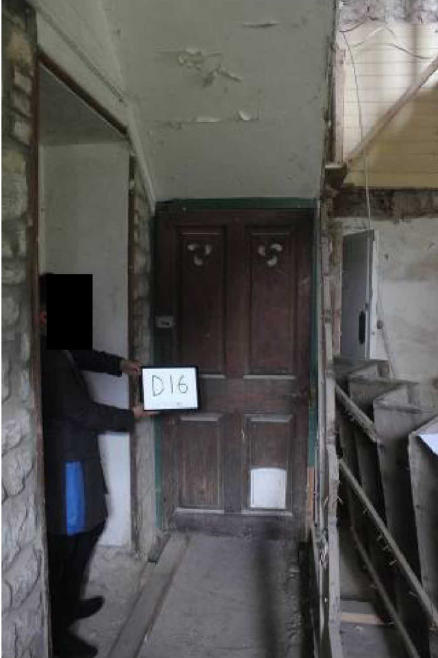
D16 S side looking along N/S passage. Note ventilation openings (and modern cat flap!) Remnants of back stairs to right
