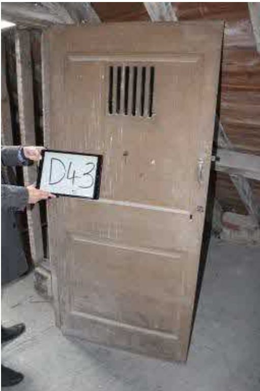
D43 outside Note ventilation slots
