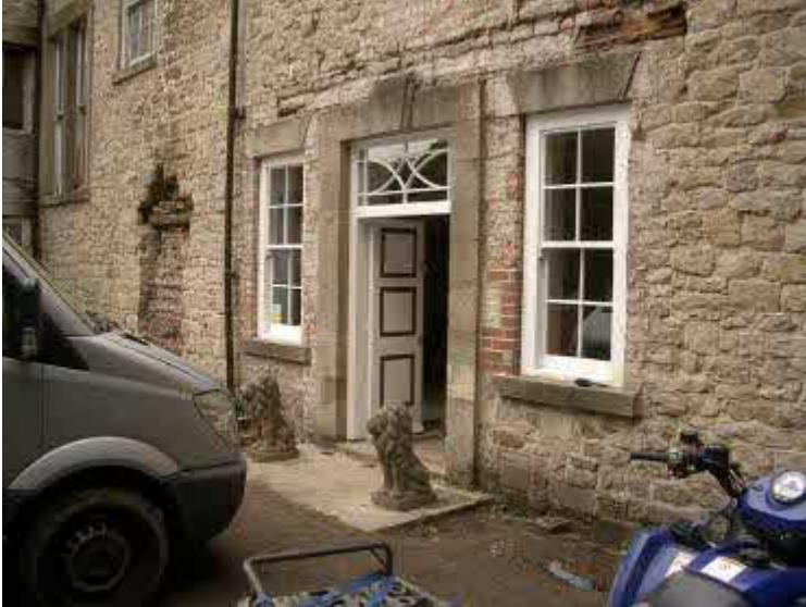
1930's entrance inserted into S wall of C19 build following removal of C19 NW range. Note blocked opening beyond in earlier fabric.
