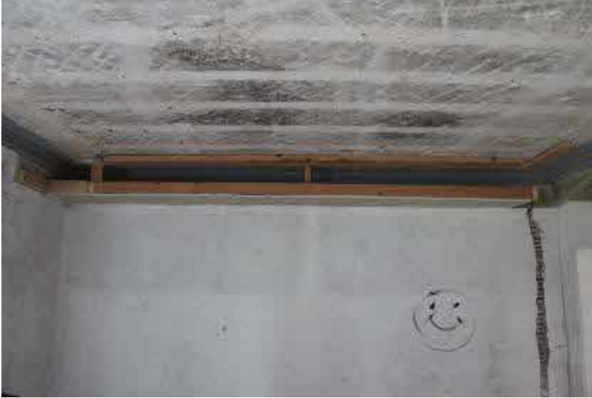
Boxed cornice E wall
