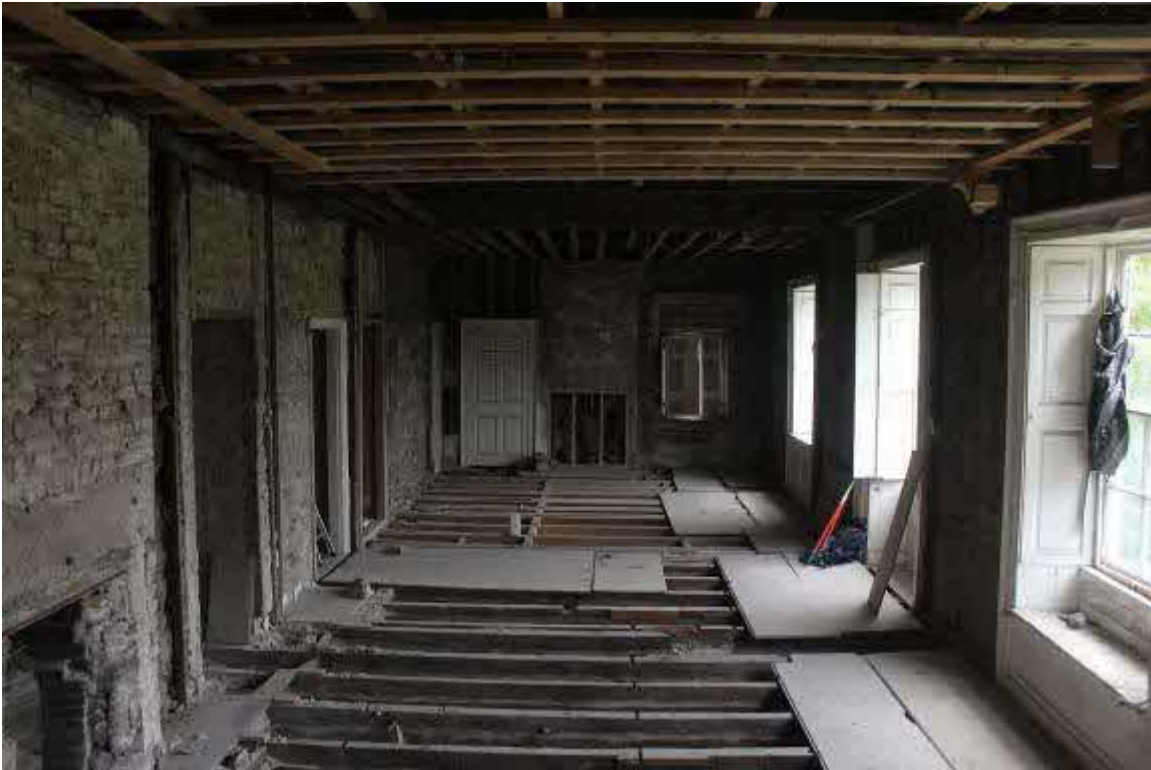
General view looking east from breach in W wall. FP8 L. foreground
