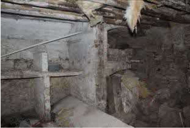
Looking SE to arched bins against S wall
