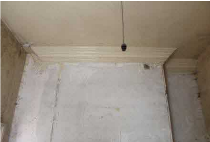
Cornice above FP2. Removed for ?1930's "Cloaks" partition (left) and continues beyond WC partition (right).
