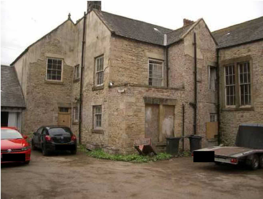
Looking from the NW to the service wing. A complex multi-period development from early C18-C20
