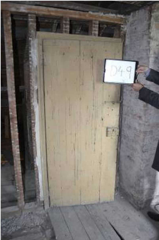
D49 room side. A much simpler and earlier (hinges) plank door, perhaps contemporary with FP13
