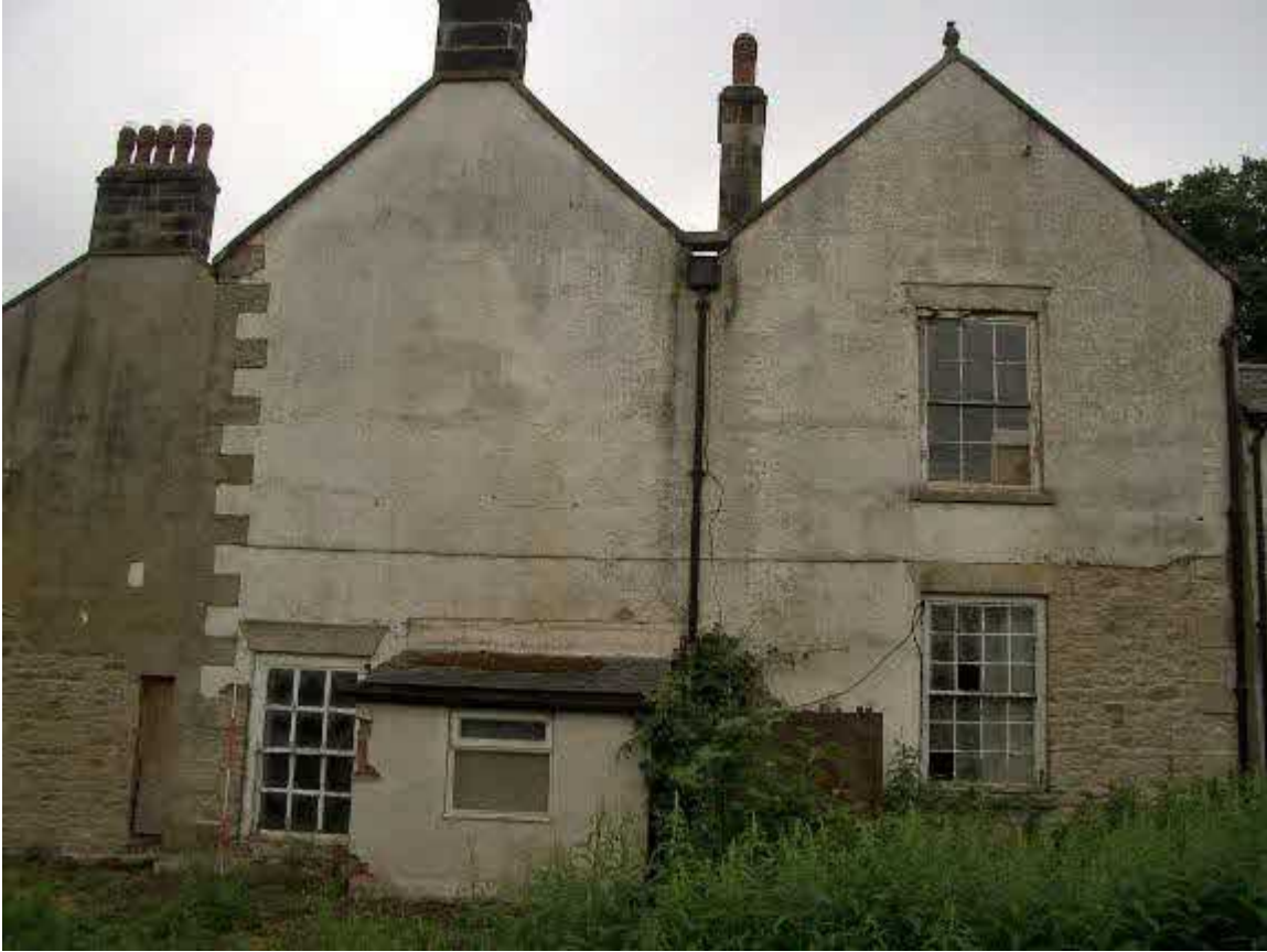
Double span block. RH GF – old kitchen W8 and W 32 above look C18 (no horns on sashes). Note stone quoins showing where render removed (right).
