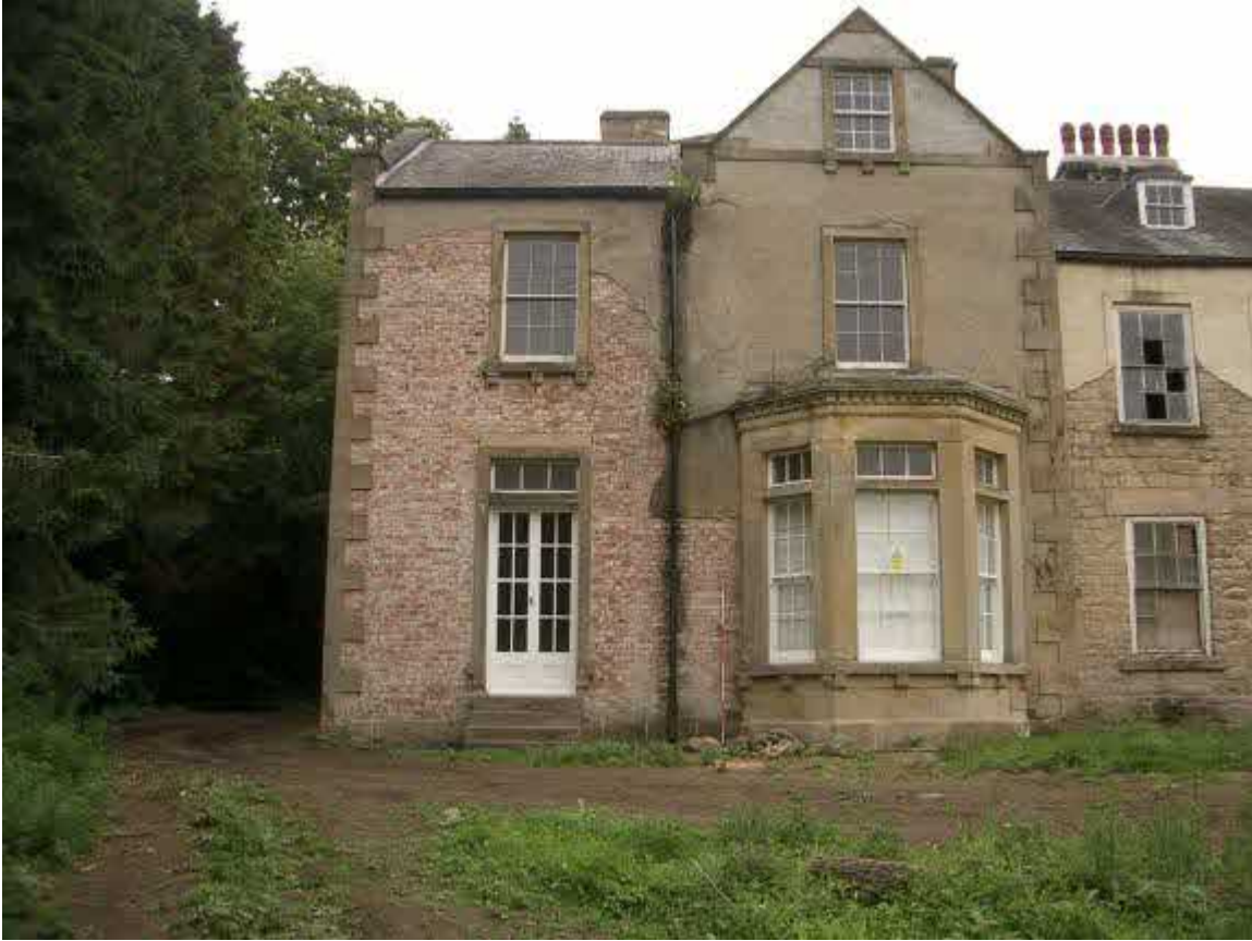
The western part of the south elevation, looking North. This 1880's addition is in brick with a Portland cement-based render, lined in imitation of ashlar
