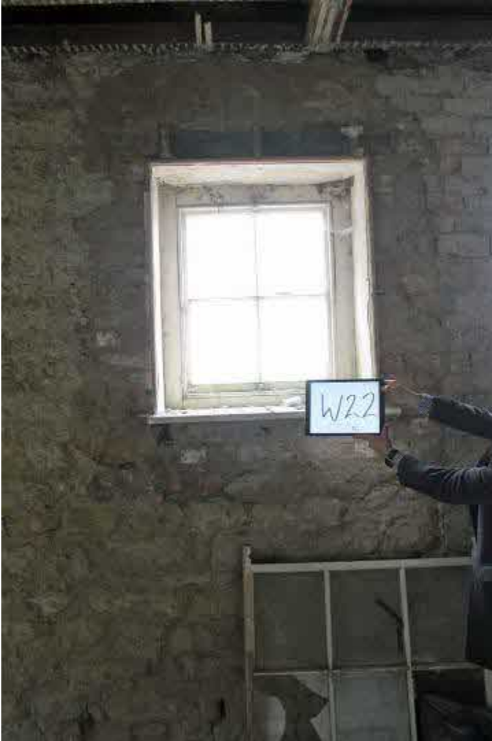
W22 inserted, with a large area of disturbance, into earlier window opening? Stonework to L and below. 1930's work to balance W 24 on re-worked N façade. Note change to brick walling to R
