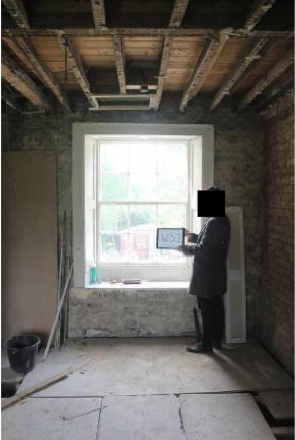
W31 Note roof access above and brick end wall to R
