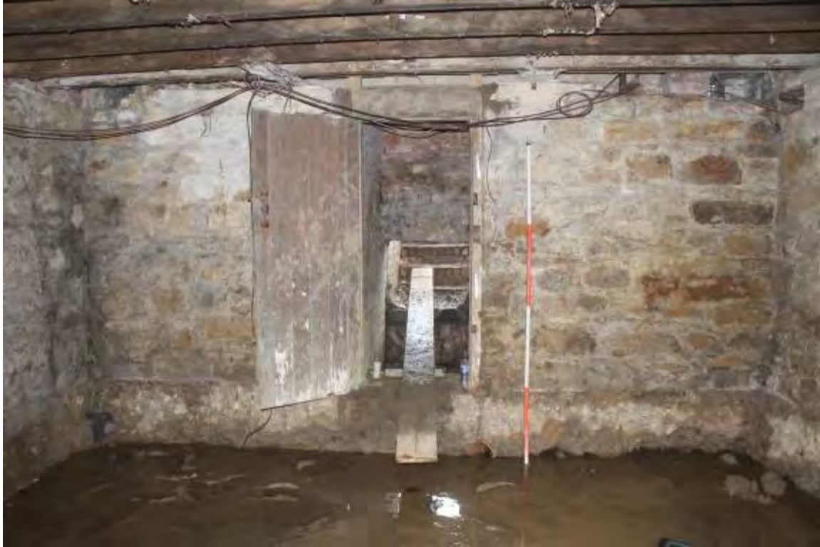
Photo 13. Door in south wall. Note substantial Victorian foundations here and drain pipe to L. of ranging rod. High level ventilation slots, top L and R
