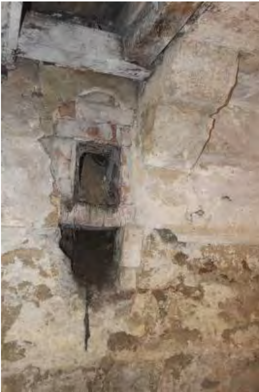
Photo 8. Vent and shute cut into cellar wall to LHS of fireplace above
