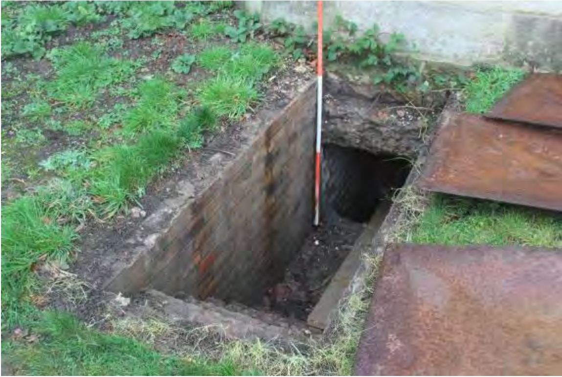
Photo 2. Steps and brick lined passage below the bay on the S. front. Note mass concrete foundation to 1880's bay and modern blocking, subsequently re-opened, behind ranging rod
