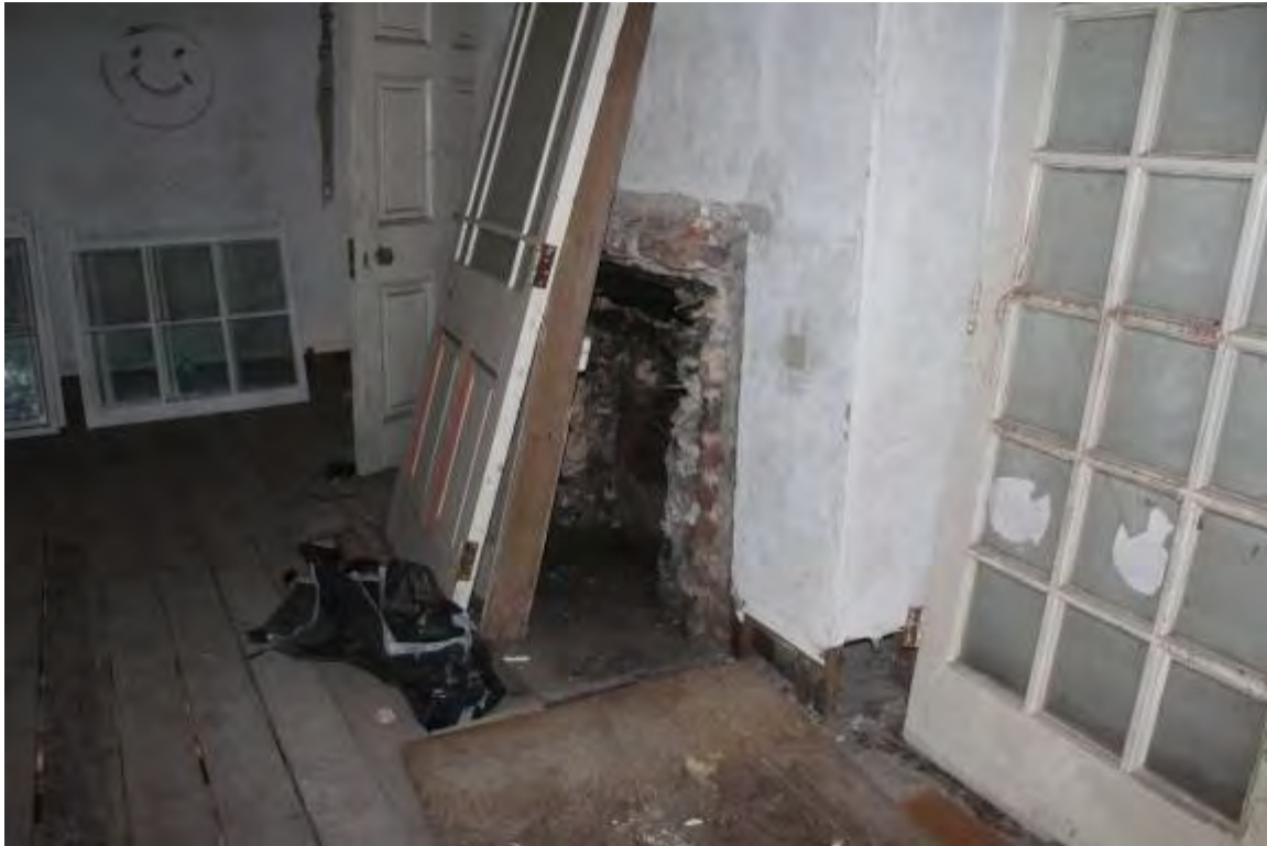
Photo 9. Fireplace and hearth in the room above
