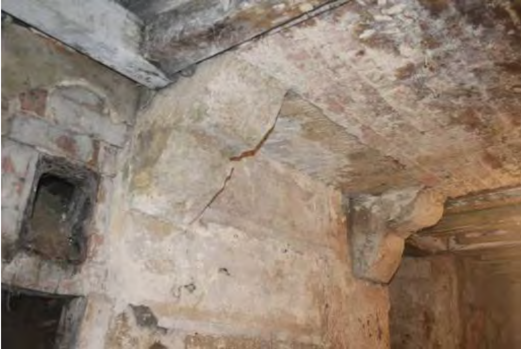
Photo 7. Corbels and brick hearth for ground floor fireplace against north wall
