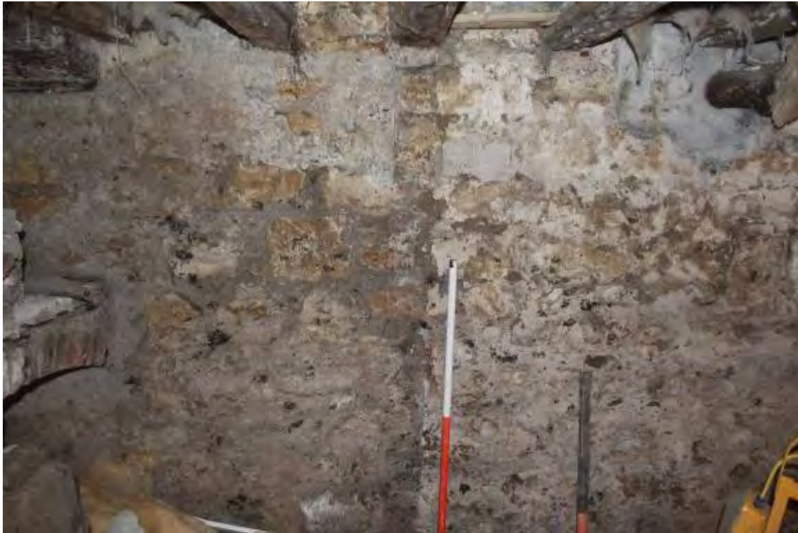
Photo 11. Traces of former N/S partition against south wall
