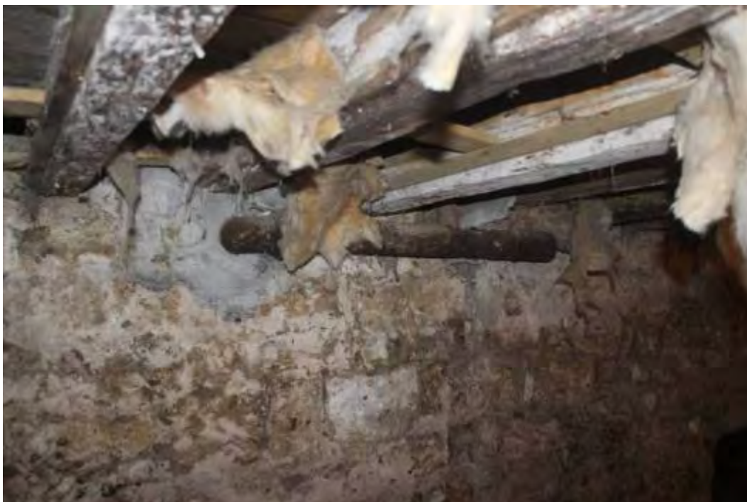
Photo 10. Four inch cast iron drain pipe against south wall of cellar
