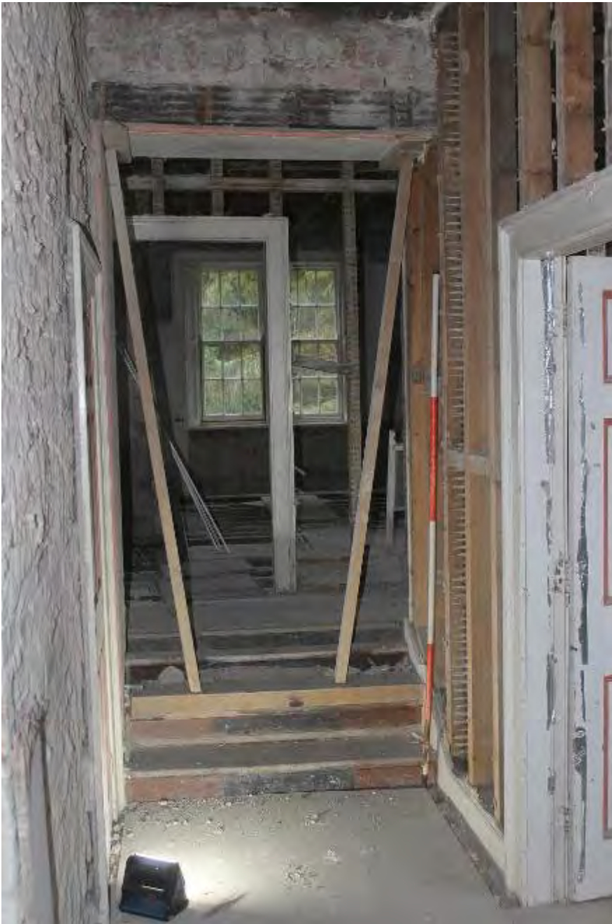
Photo 19. View looking west along landing. Wallpaper surviving behind studwork partition adjacent to ranging rod. Note timber props resting on second step and brick relieving arch over timber lintel above 1880's opening through earlier gable wall
