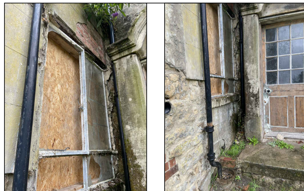
External view of window W11
