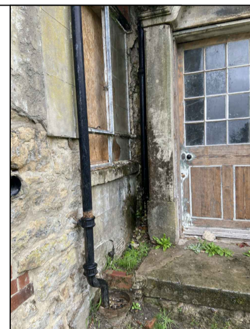
External view of window W11 and door D5
