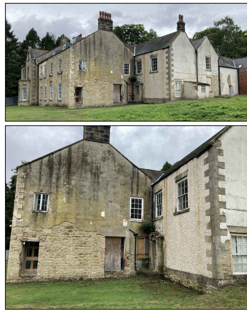
External views showing east elevation
