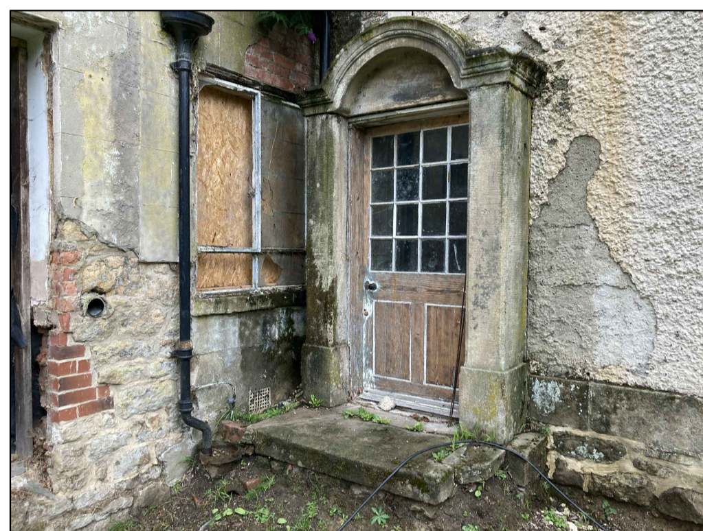
External view of window W11 and door D5
