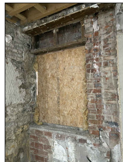
Internal view of window W11
