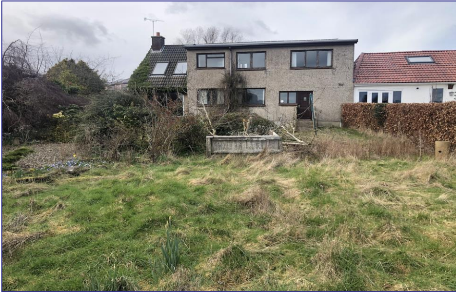
Photographic Plate 11 – Back garden and dwelling looking west.
