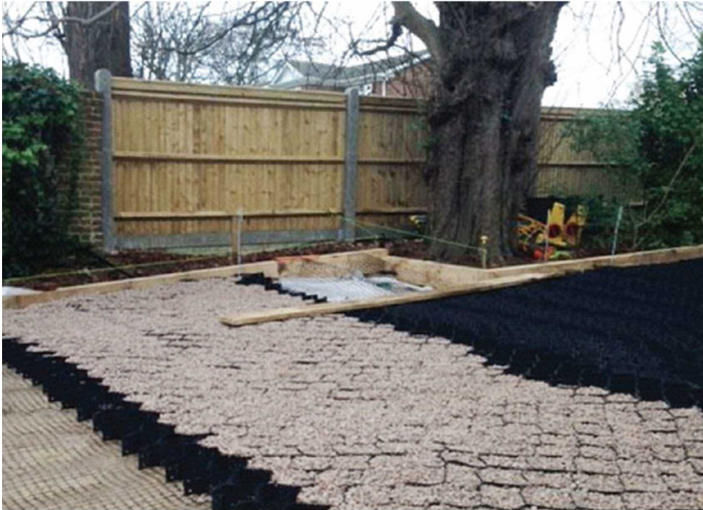
Figure 1: Example of installation of cellular confinement system within RPA.
