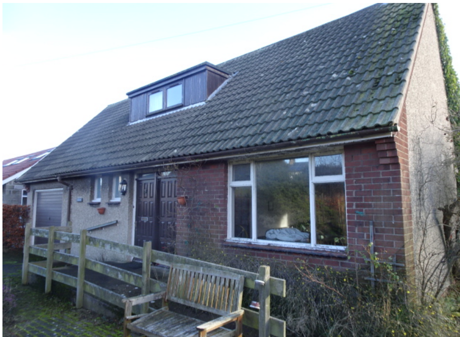
Front elevation showing dormer window
