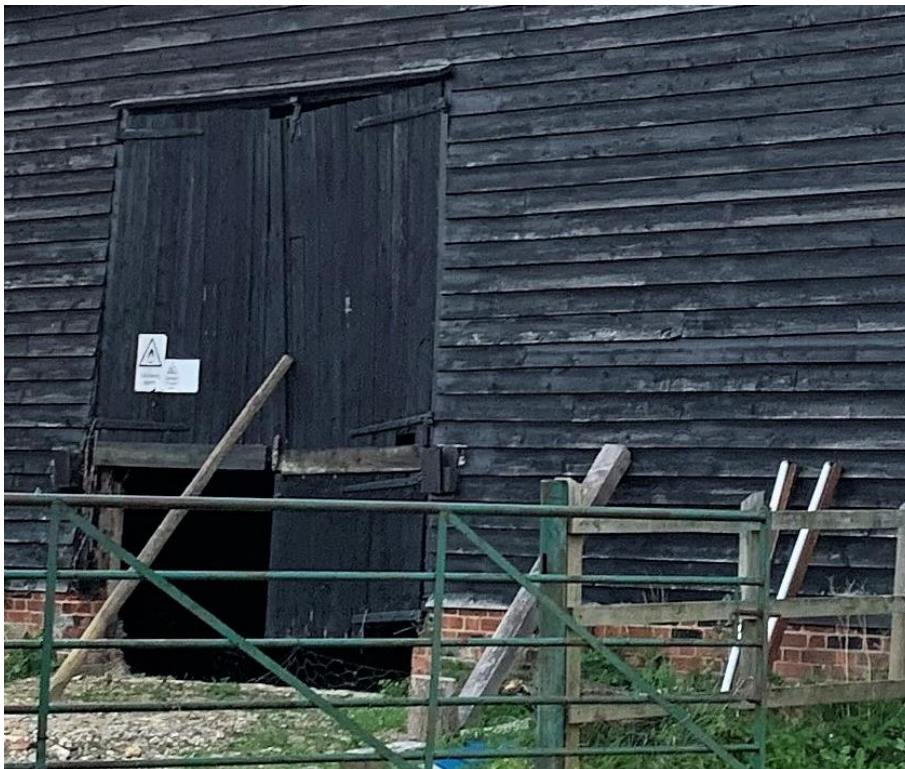
Plate 3.1: Western elevation of B2 – (Photo: 07/09/21 – O. Robson)
