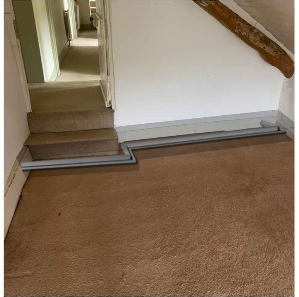
06. Bedroom 4 Proposed - plumbing to run along the same route on floor level and boxed in. Existing step to be suitably extended.
