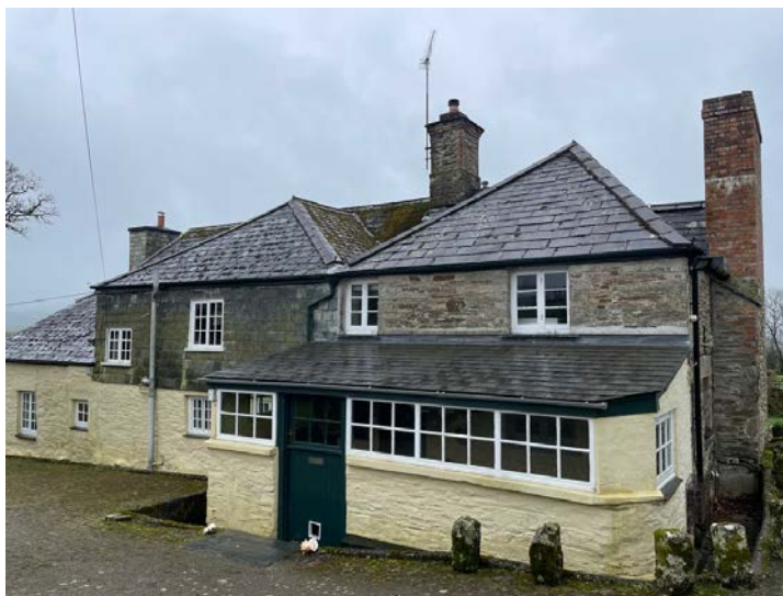
Figure 1&2: The south west front and north east rear of the farmhouse
