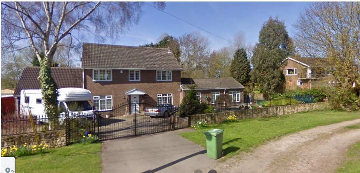
Fig.6: Two storey brick-built dwellings facing east on to the village green
