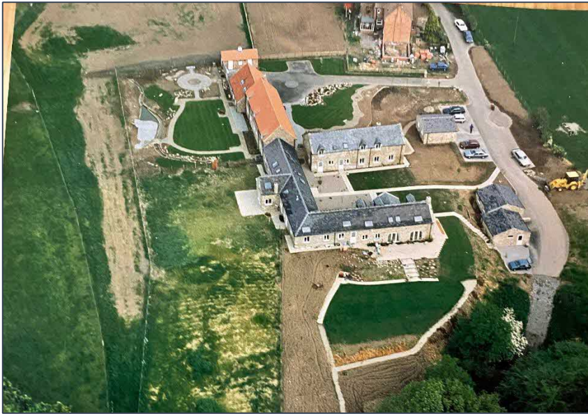
Photo 5 Conversion works in progress
