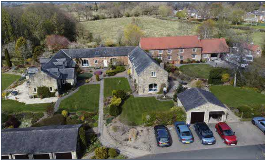
Photo 6 The completed conversion today
