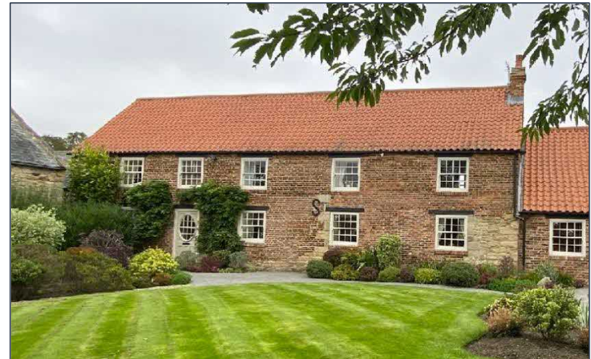
Photo 3 Front south elevation today
