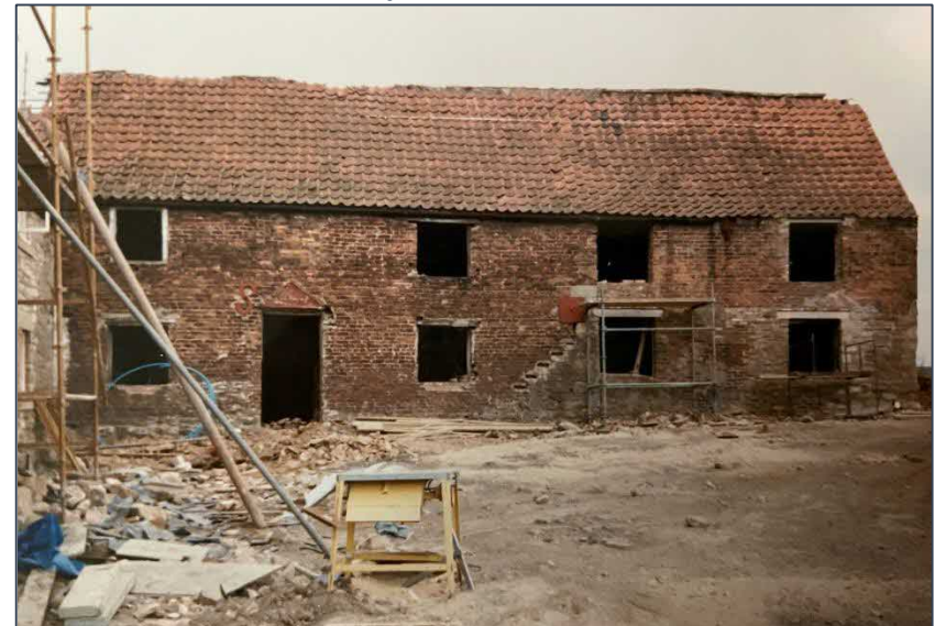
Photo 4 Front south elevation prior to conversion from pigsty to dwelling
