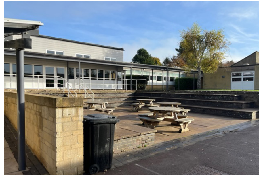
2 - View across amphitheatre to dining & 6th form common room
