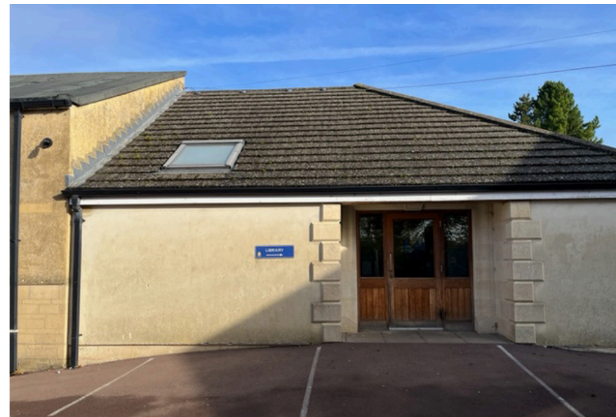
5 - Entrance into library block
