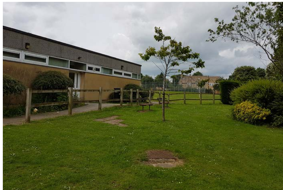
4 - View of existing sixth form block
