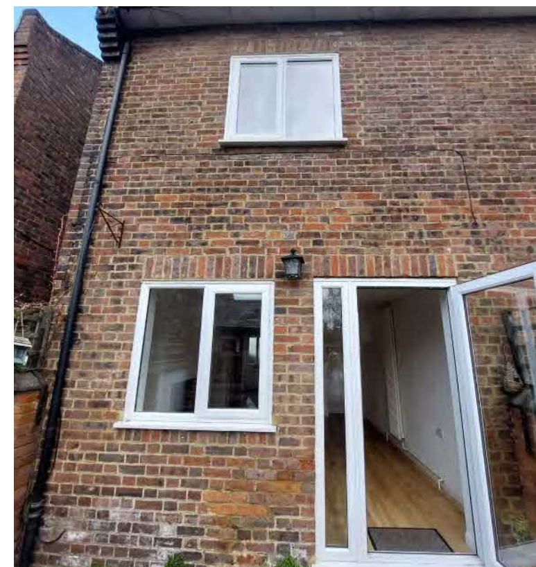
Figure 4.4 Rear elevation of 1 Royal Court.
