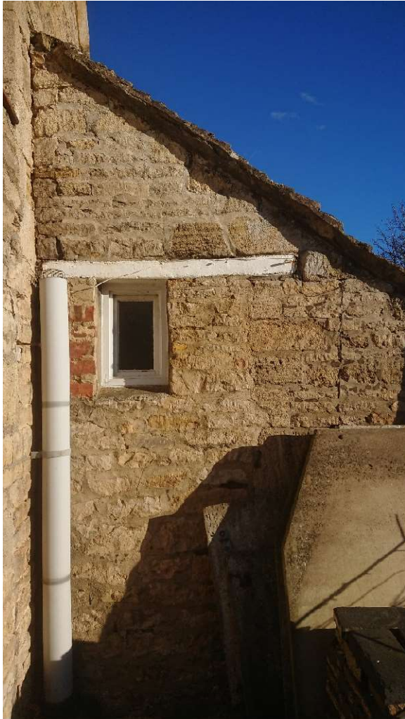
Photo 13: Blocked up Lean-to Doorway
