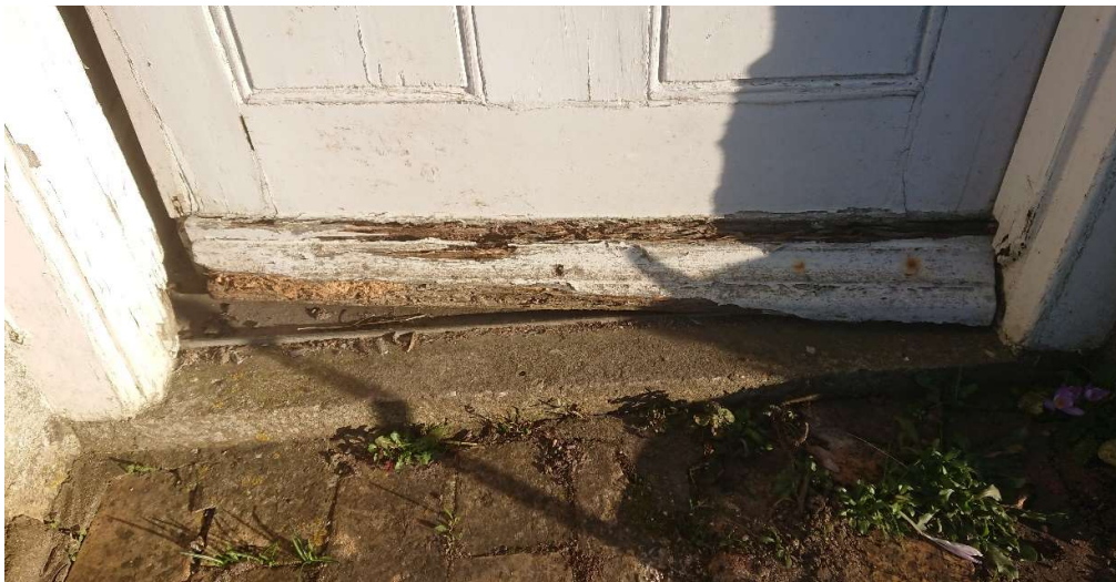
Photo 6b; Front Door's Concrete Threshold
