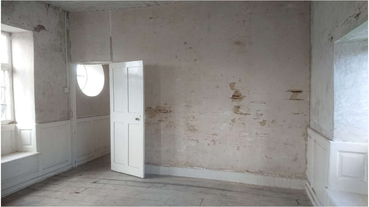
Photo 10a: Schoolroom Victorian Partition
