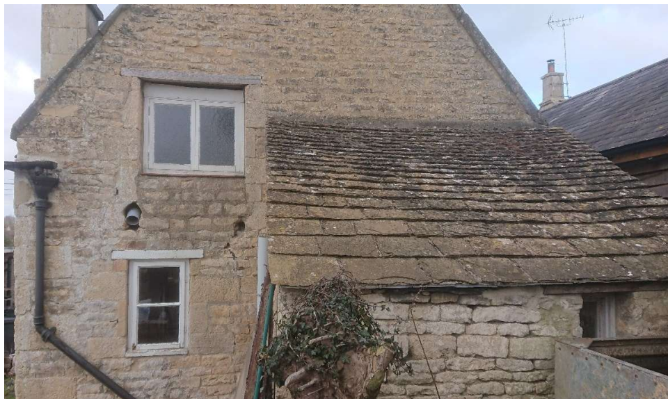
Photo 8: South Gable of Lower Range and Lean-to Roof
