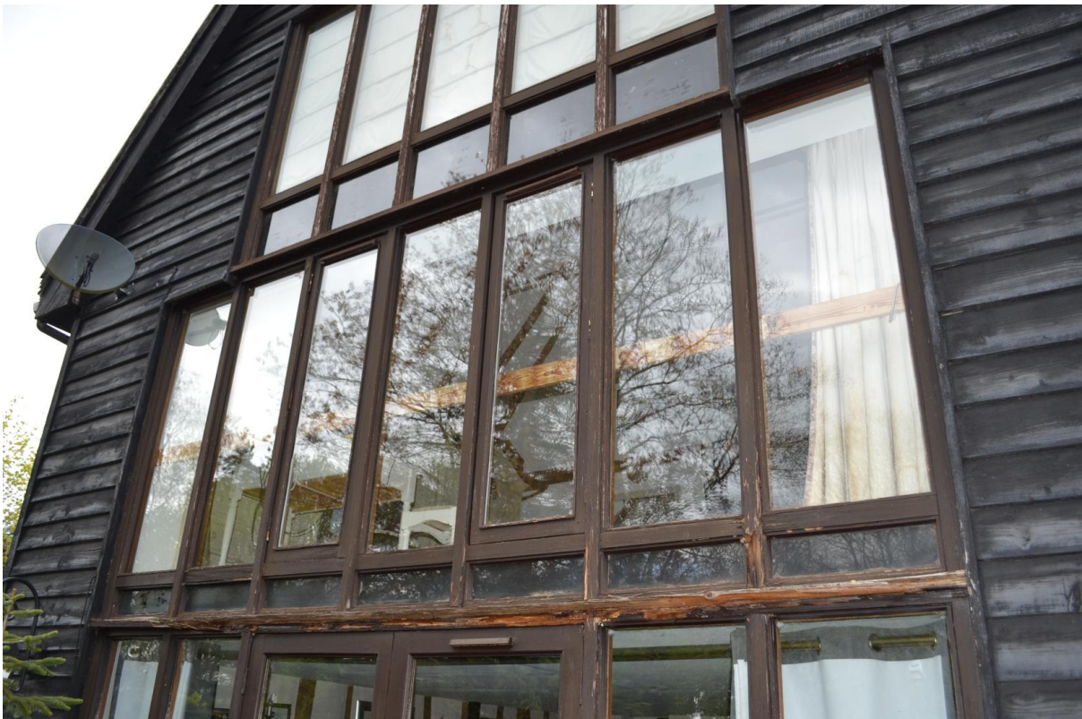
Plate 2 - Note the full height windows, with no balustrade to the barrier.
