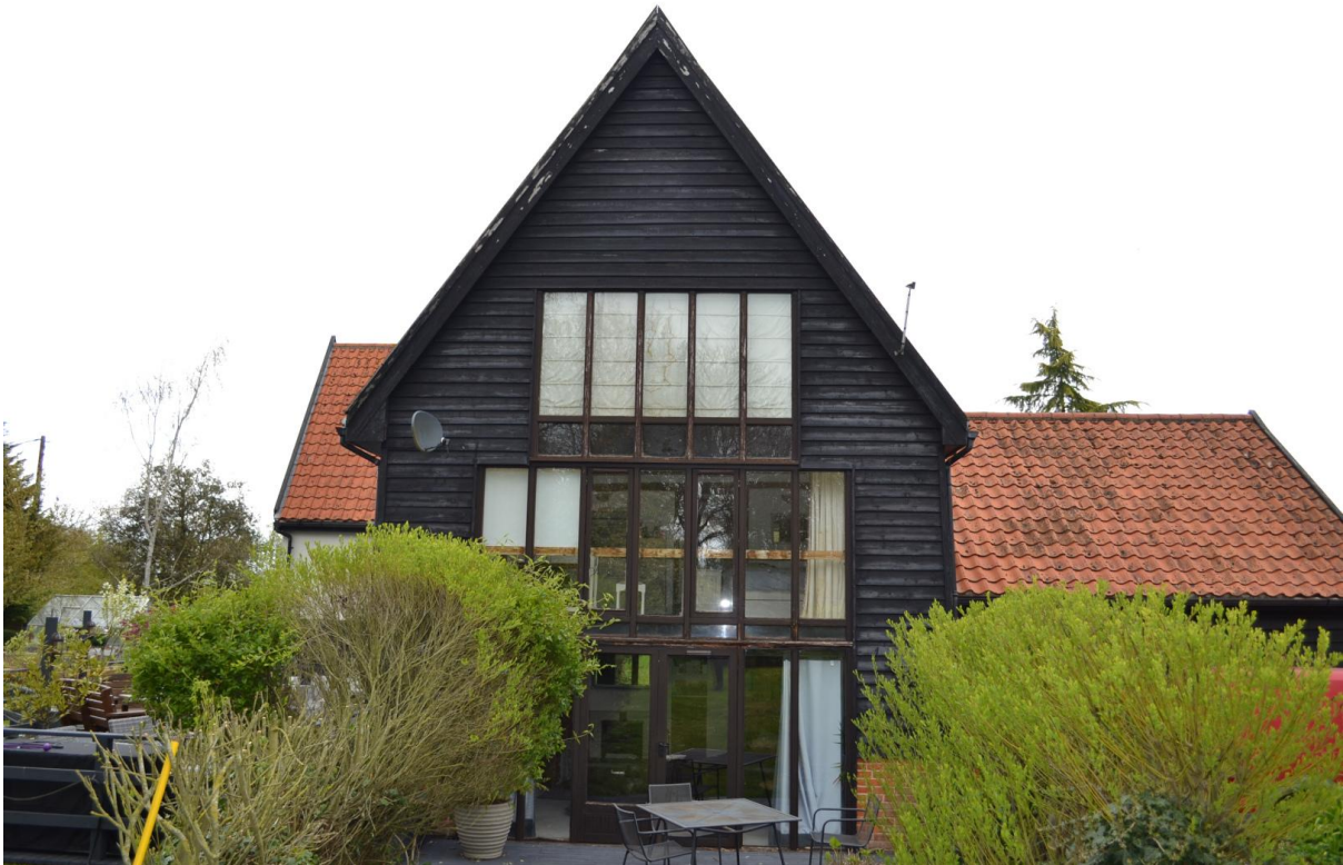
Plate 1 - Gable hosting glazed screens to be replaced
