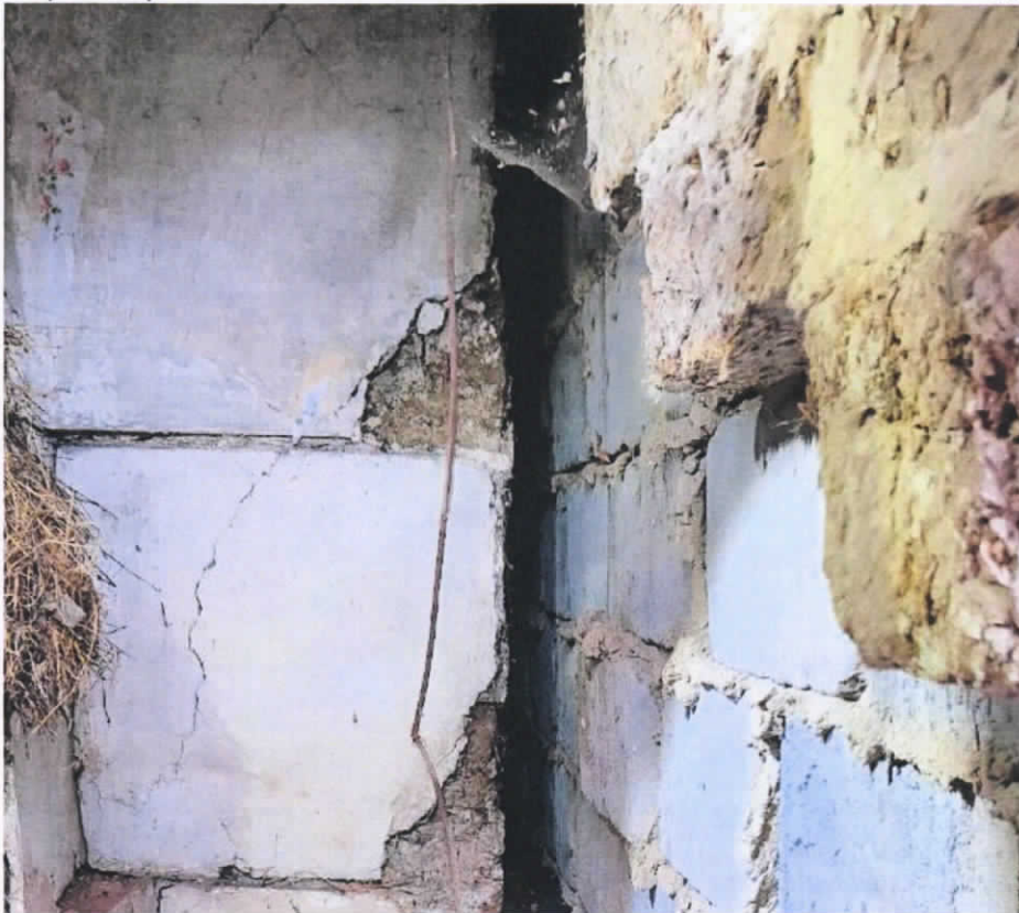
The collapsed wall (purple arrow) leaves either some or all the brick plinth in place. The east elevation brick plinth is wider than the west elevation. That could indicate past works to protect erosion of the wall.
