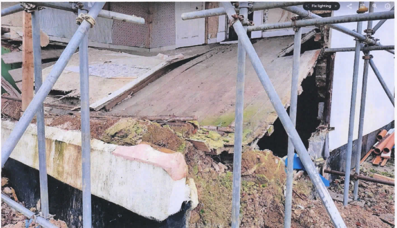
The collapsed wall (purple arrow) leaves either some or all the brick plinth in place. The east elevation brick plinth is wider than the west elevation. That could indicate past works to protect erosion of the wall.
