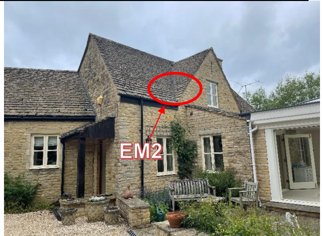
Photograph 8: South and eastern elevation of the right-wing.
