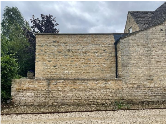
Photograph 11: Northern elevation of right-wing and extension.
