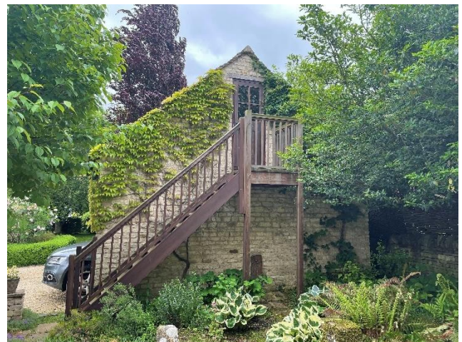
Photograph 4: Western elevation of garage.
