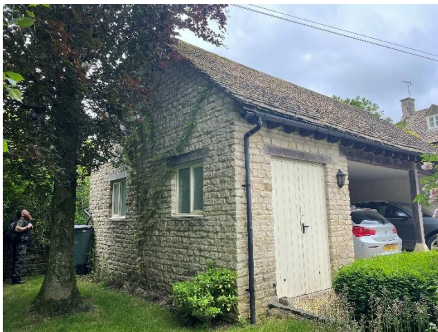
Photograph 3: View of northern and eastern elevation of garage.
