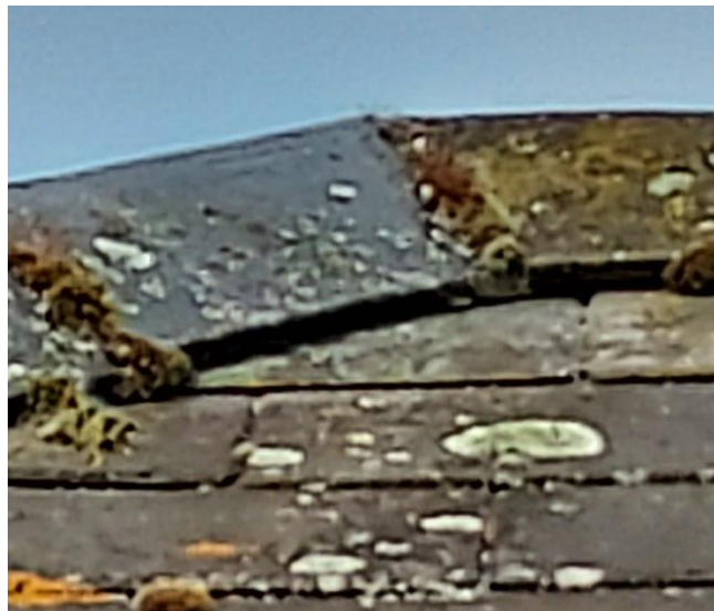
Photo 8: Ridge tile access
