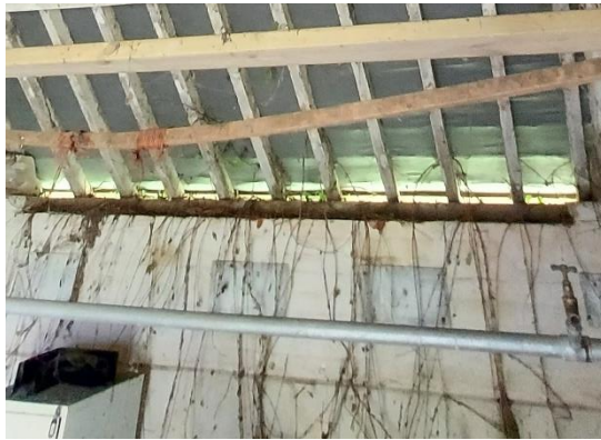
Photo 10: Access under soffits
