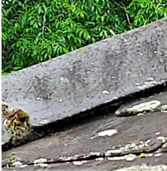
Photo 9: Access at a hip ridge tile
