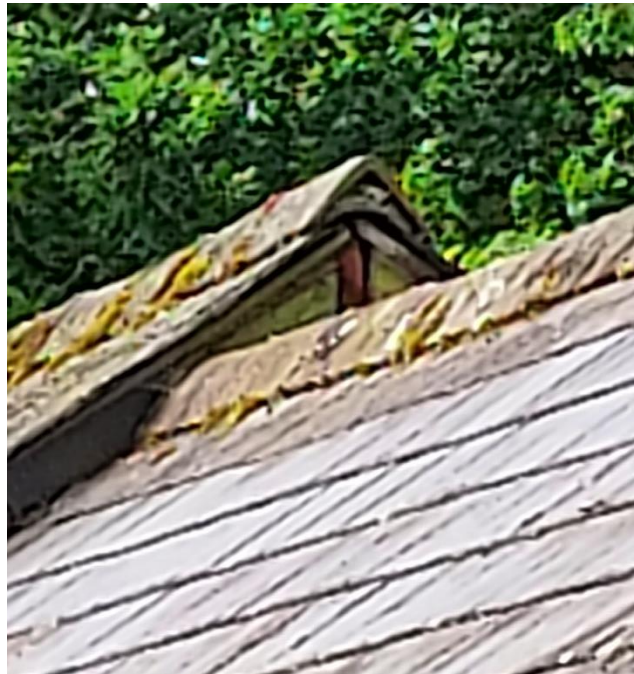
Photo 7: Access at the ridge tile where two sections of roof meet
