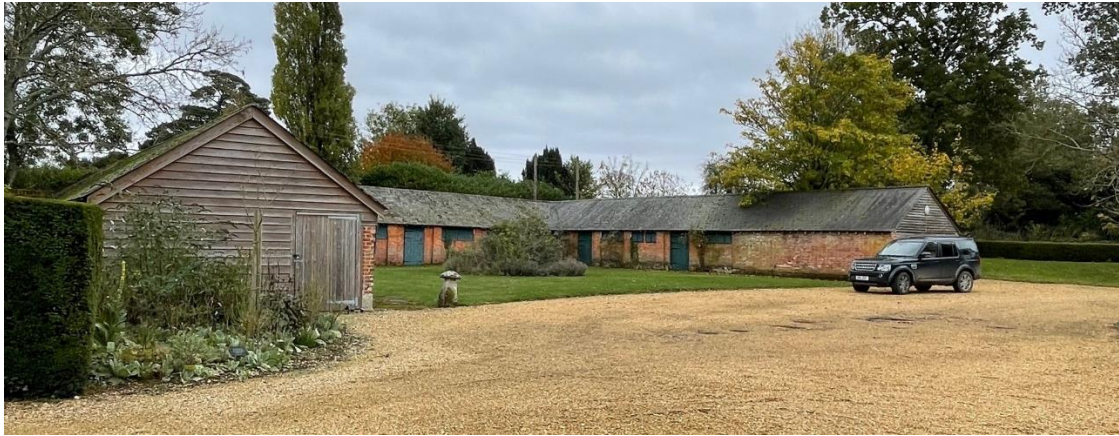
Photo 1: The building from the north-west
