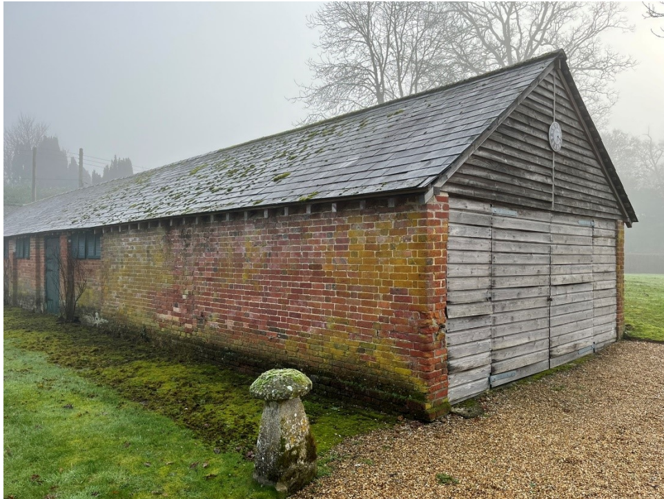
Image 5: Gable end of stable with timber cladding visible.
