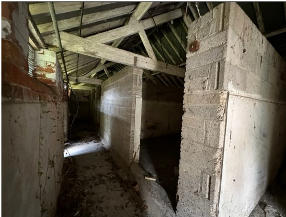
Image 14: Internal view of the stable building with block and concrete evident.
