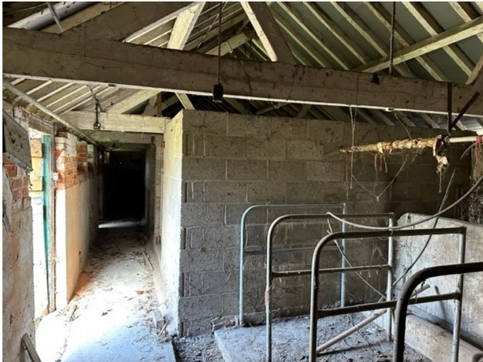
Image 13: Internal view of the stable building with block and concrete evident.
