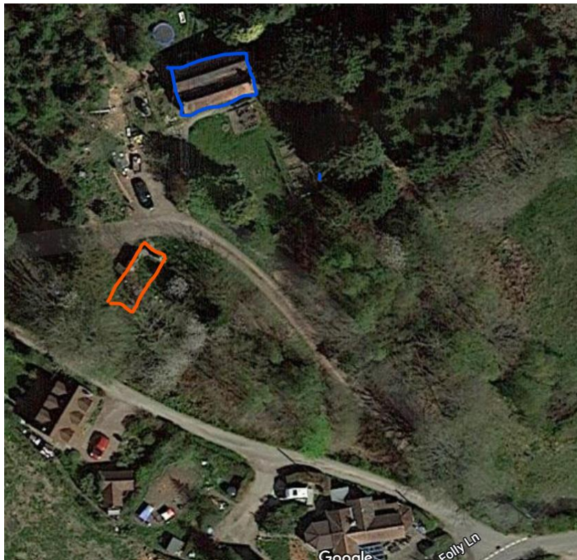
Figure 1: Google Earth screen shot with Folly marked in Blue and barn marked in red.
