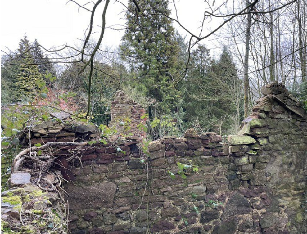
Image 3: view east across internal dividing wall
