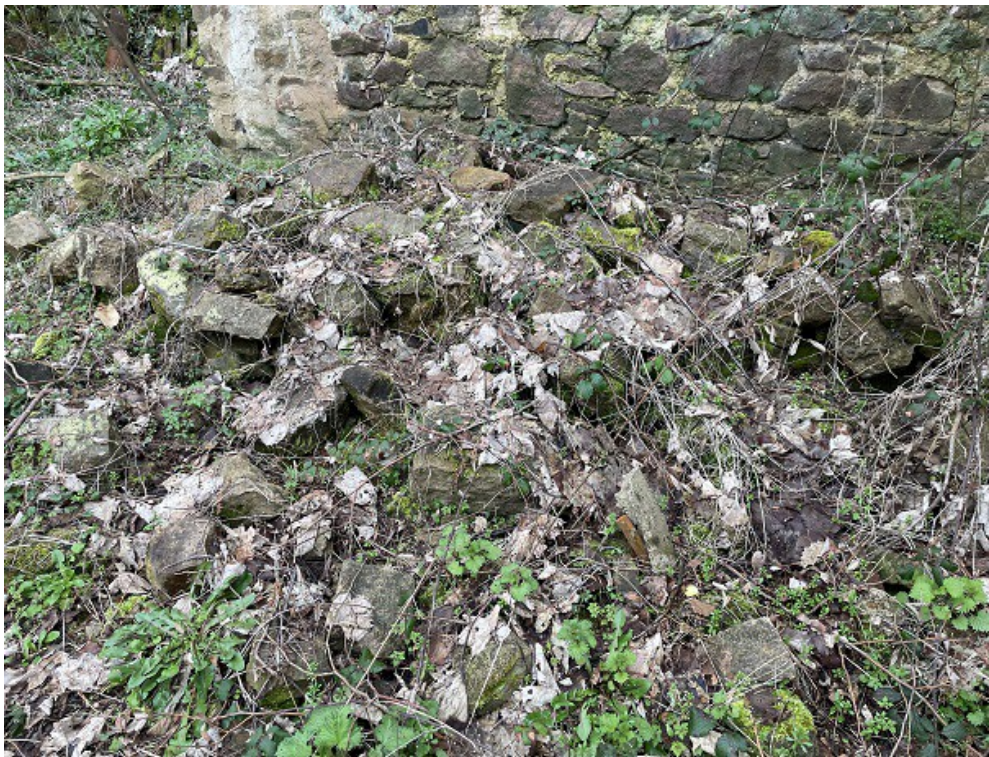
Image 8: stone rubble pile inside the structure (target note 1)
