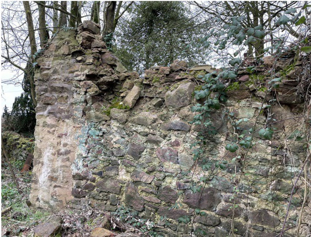
Image 4: inside view west gable end wall
