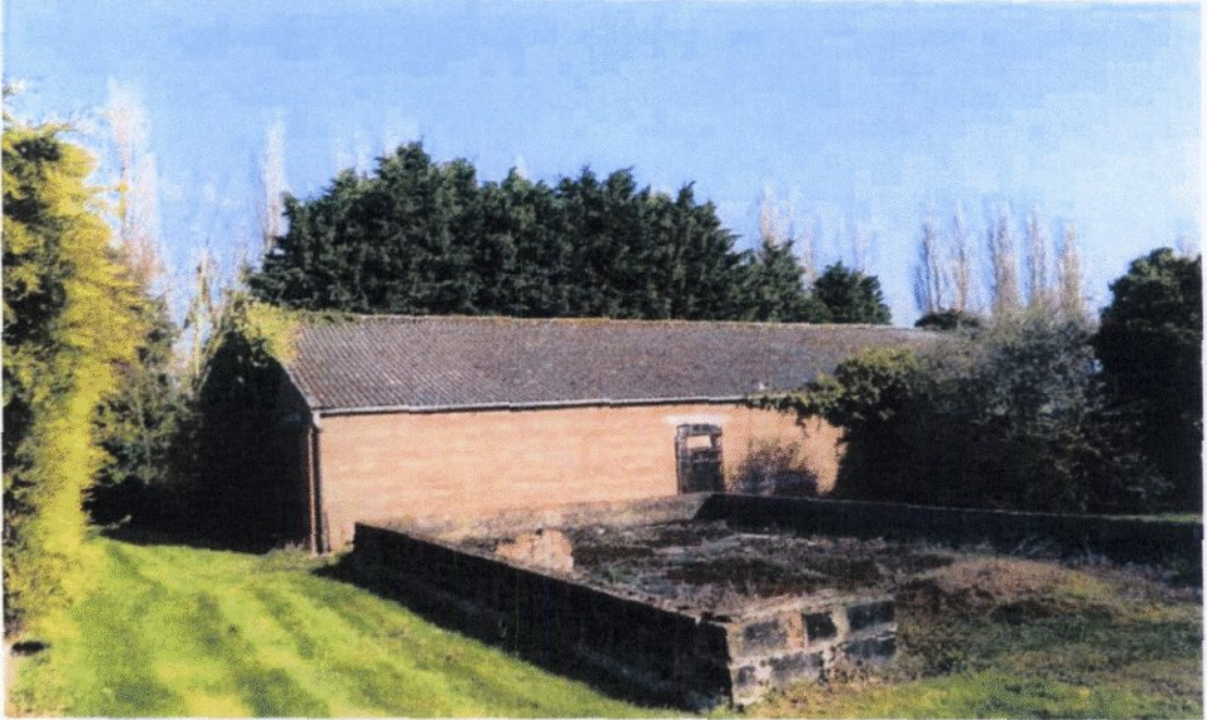
Barn 2003 (Moors Lodge Farm North)
