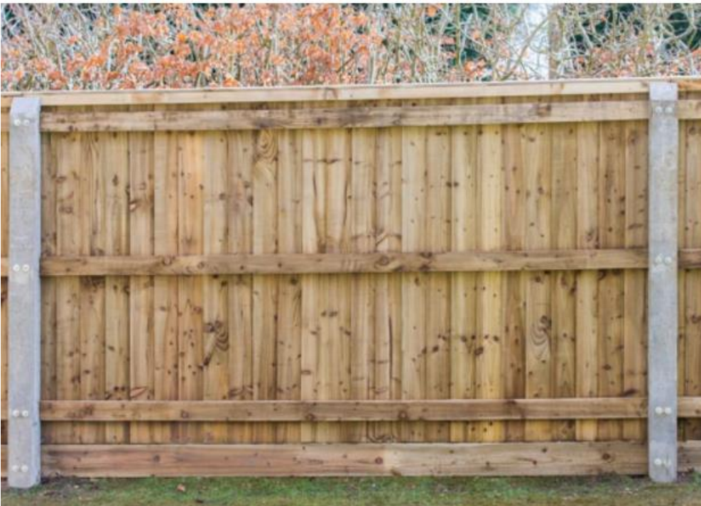
Timber close board fence with concrete posts.
