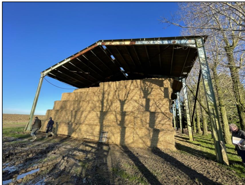
Figure 2.6 Existing Straw Barn, Western Elevation
