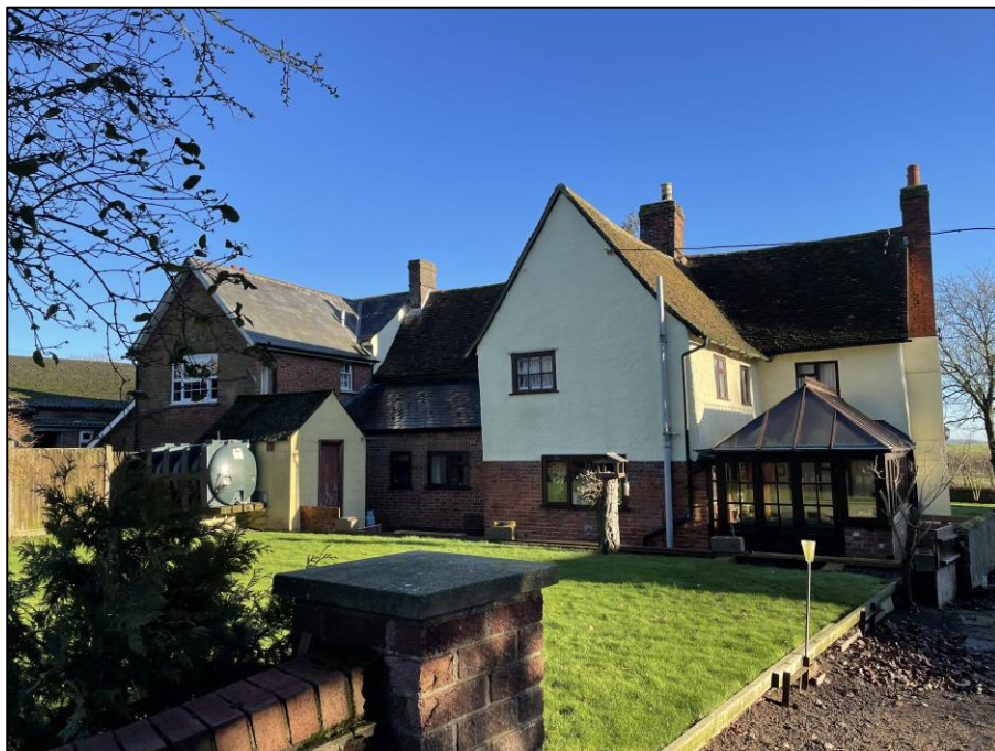
Figure 2.4 Slate Hall Farmhouse From The Rear Elevation, Grade II Listed
