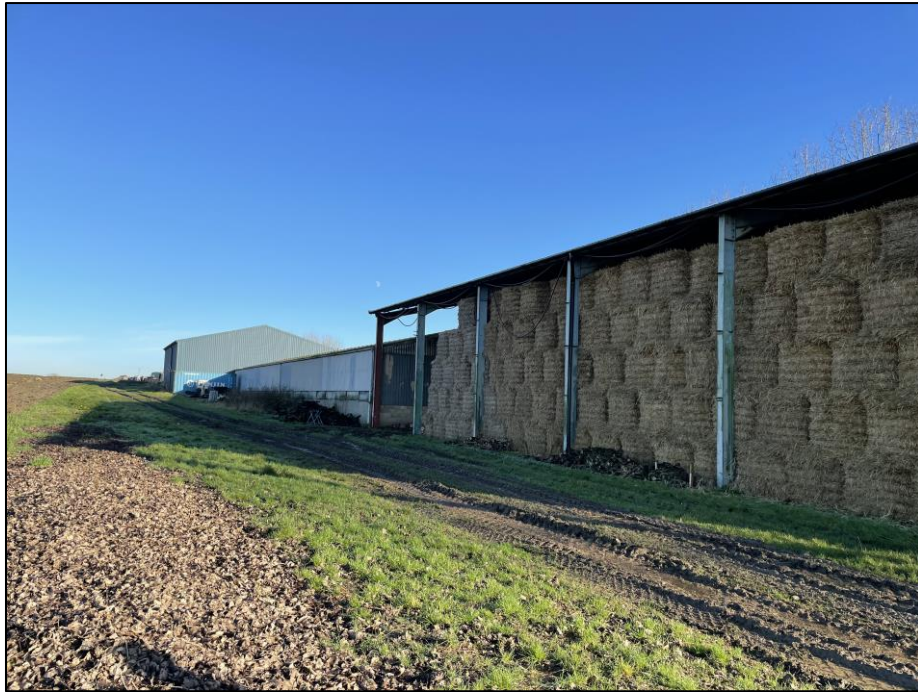
Figure 2.7 Straw Barn And Adjacent Buildings
