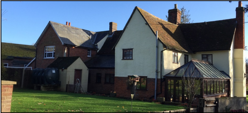
View of rear of Slate Hall Farmhouse.
