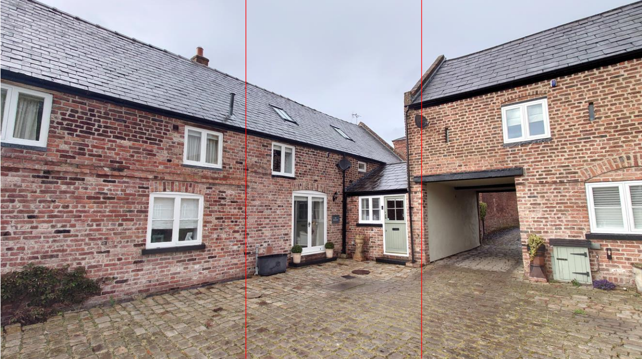
View north from courtyard
