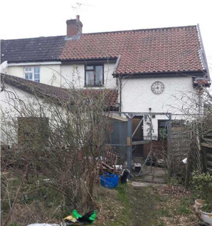
Photo 2. North face of Building 1
