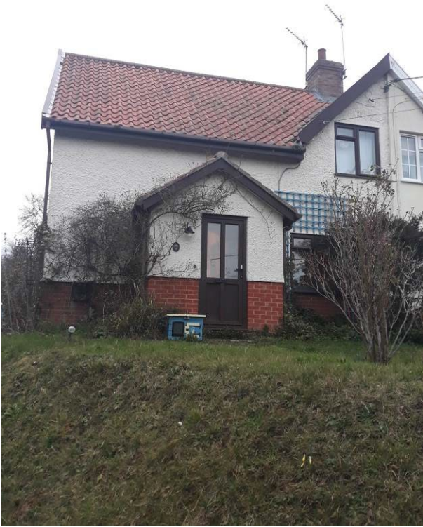
Photo 1. South face of Building 1 .
