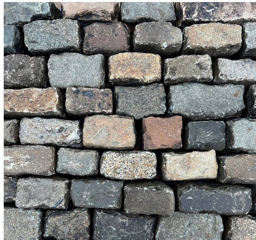
Granite setts (to road Margin
