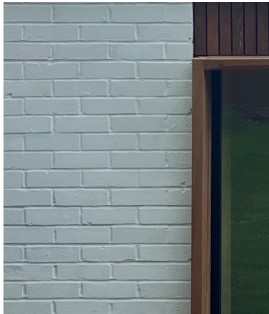
Existing brickwork render to the rear to receive a coat of Zinsser exterior breathable masonry paint to the color reference RAL 9010. See against European Oak.
