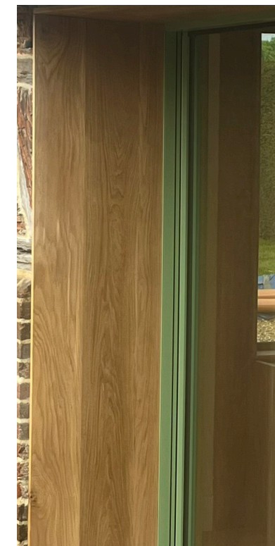
(Left) Cortizo aluminium slimline sliding doors and fixed windows (middle), with PPC coated aluminium framing color to match Lick 07. European Oak surrounds (middle). European Oak framed entrance door (right)
