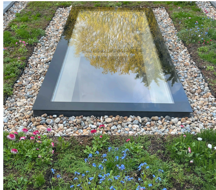
New wildflower roof, with gravel margin and Neo Roof-light (rear extension)
