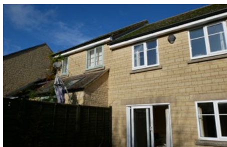
Fig.2 Site of proposed rear extension to copy form of the extension at 25 which is visible here.
