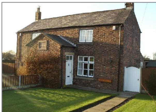
Two semi-detached houses on Altcar Road (Originally a School House)
