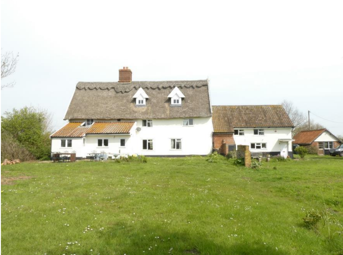
Photo 5 , south aspect of building one, looking north.
