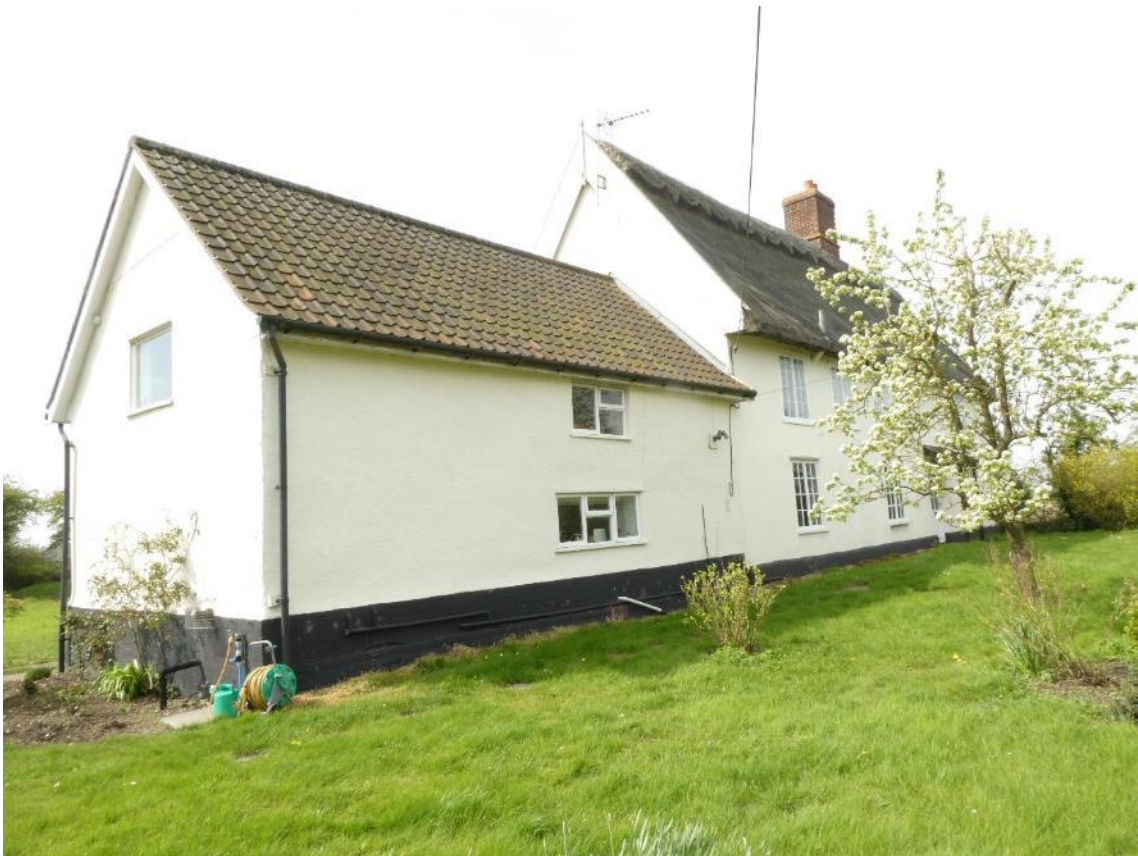
Photo 6 , north and east aspect of building one, looking southwest.
