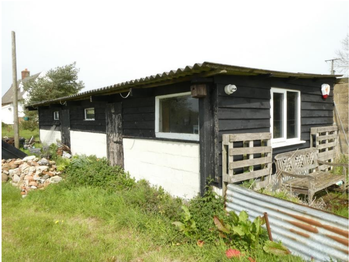
Photo 8 , east and south aspects of building two, looking northwest.
