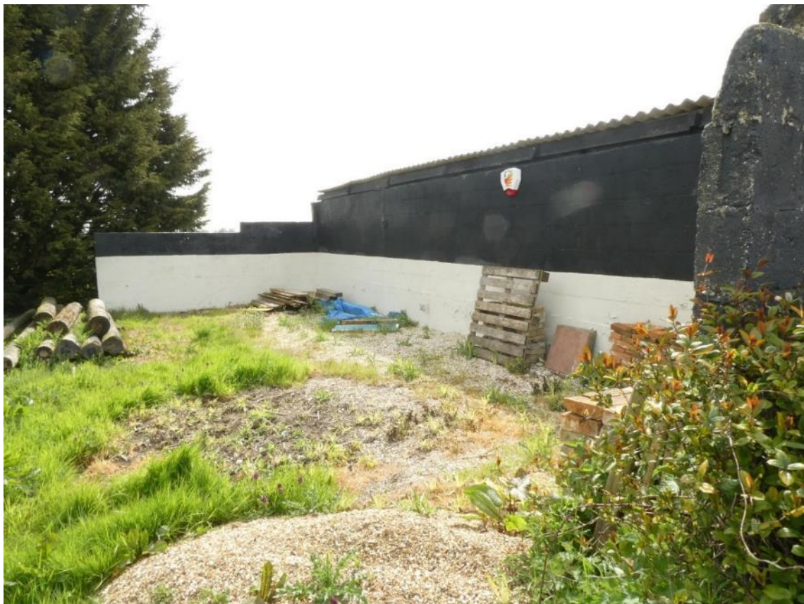
Photo 7 , north aspect of building two, looking southeast.
