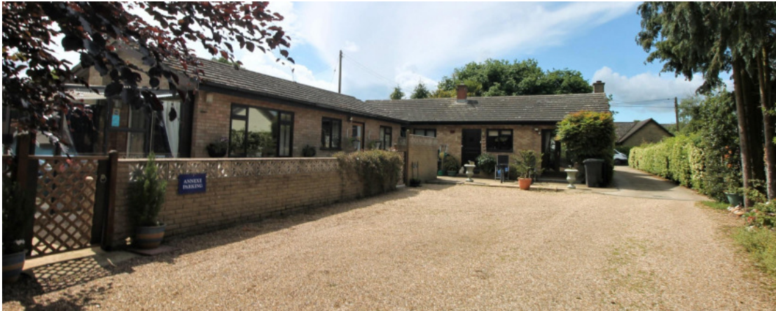
Existing Spooners Main Bungalow and The Annex
