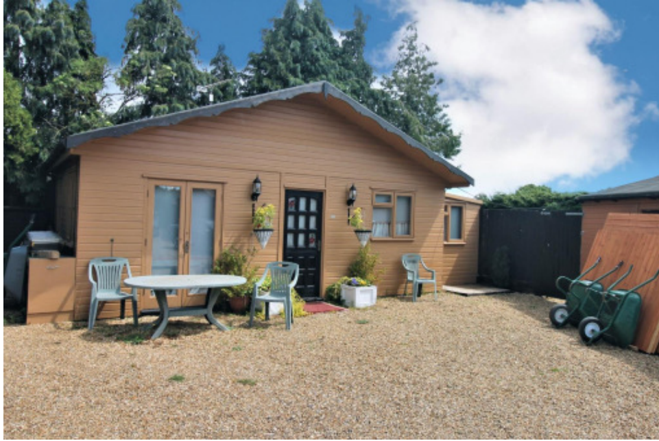
Existing Building to be Replaced
