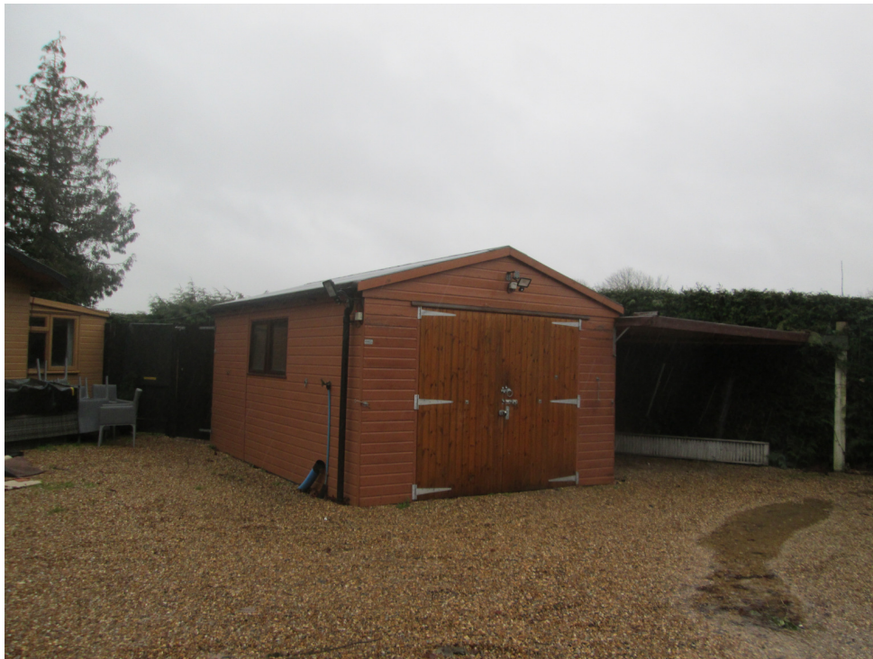
Existing Garage to be Dismantled
