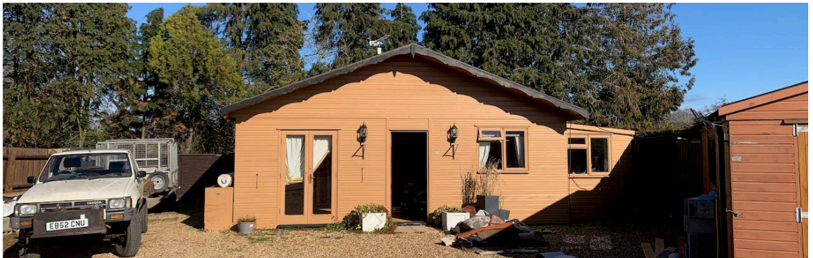
Photograph 1. Bungalow – south aspect
