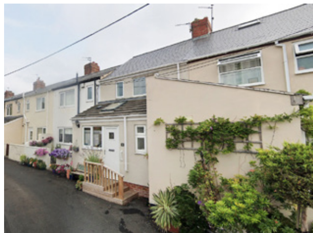
Older Terraced Row, Pond Street
