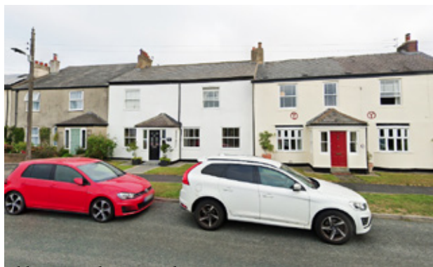
Older terraced units, High Street
