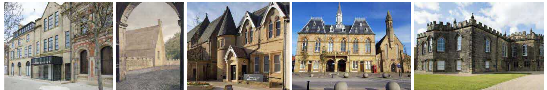
Fig. 76 Examples of stone clad buildings in the town
