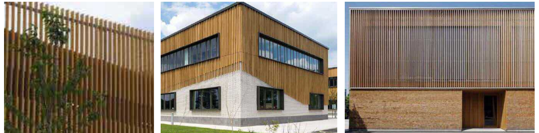
Fig. 80 Design Inspiration - examples using timber cladding at high level above solid masonry bases
