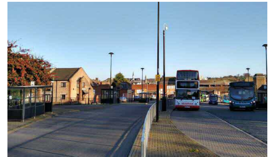
Fig. 15 Clayton Street Properties looking west
