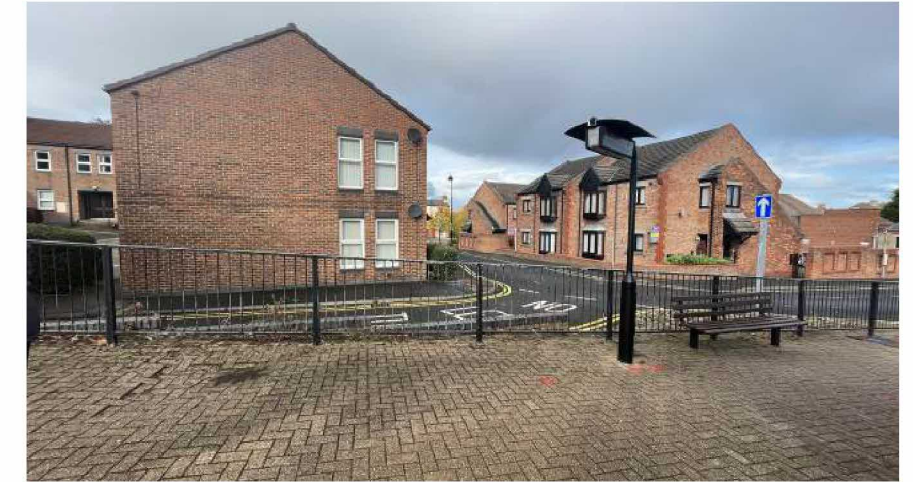
Fig. 20 Existing residential properties facing the site
