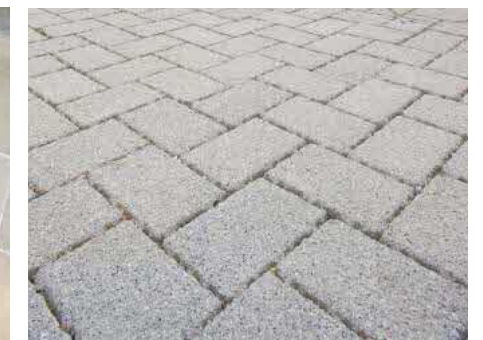
Fig. 59 Permeable blocks parking bays
