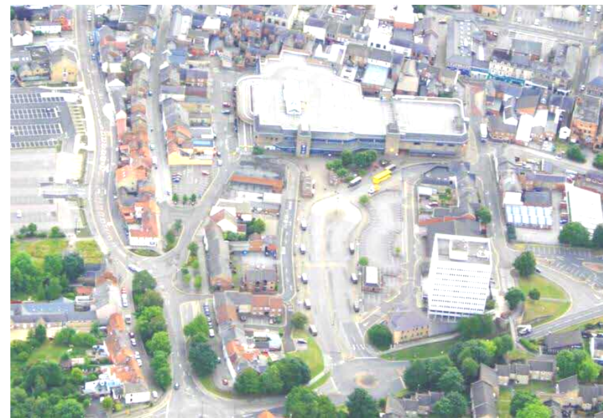
Fig. 71 3D aerial of existing site
