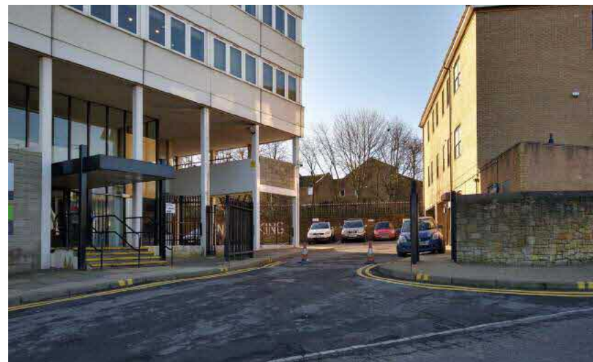
Fig. 16 Saddler Street Properties looking south west
