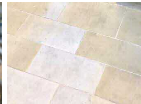
Fig. 58 High quality stone pedestrian paving
