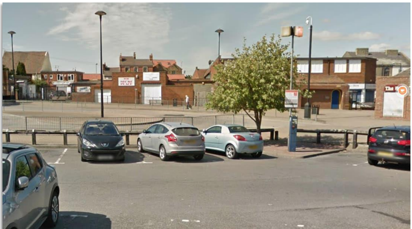
Figure 2 Existing lighting have generic lighting optics, a number have limited control – no dimming or group dimming is employed.
